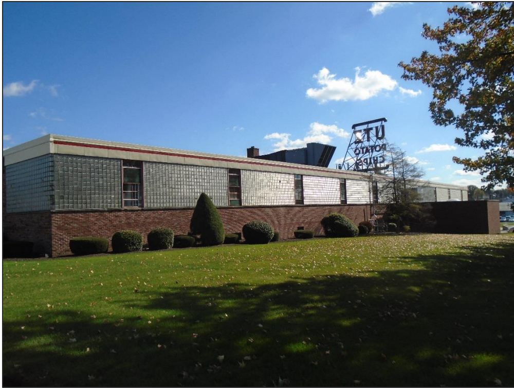
Photograph 31: The west elevation of the ca. 1949 Utz building, showing the band of glass block glazing with interspersed steel windows; looking southeast.
