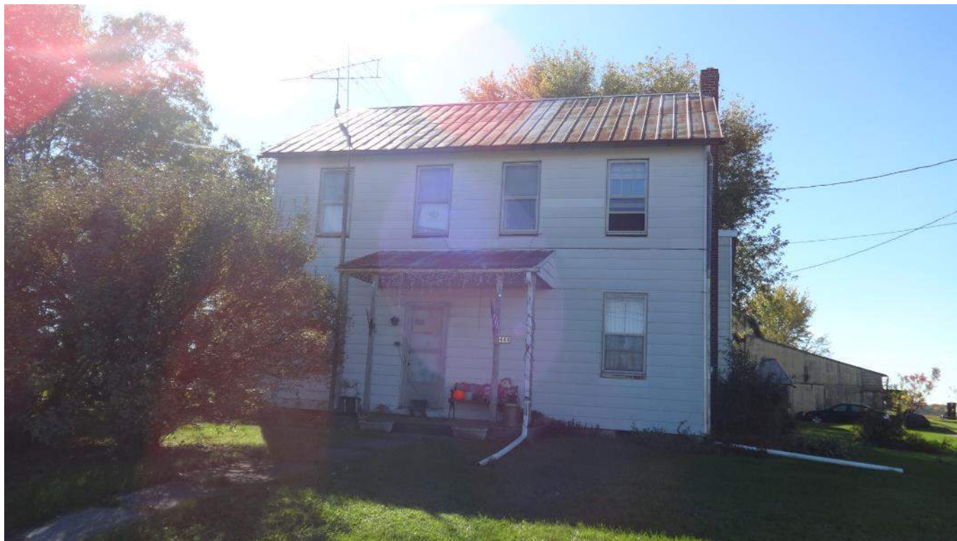
Photograph 1 – Façade (northeast elevation) of the Poist Farm dwelling; looking southwest.
