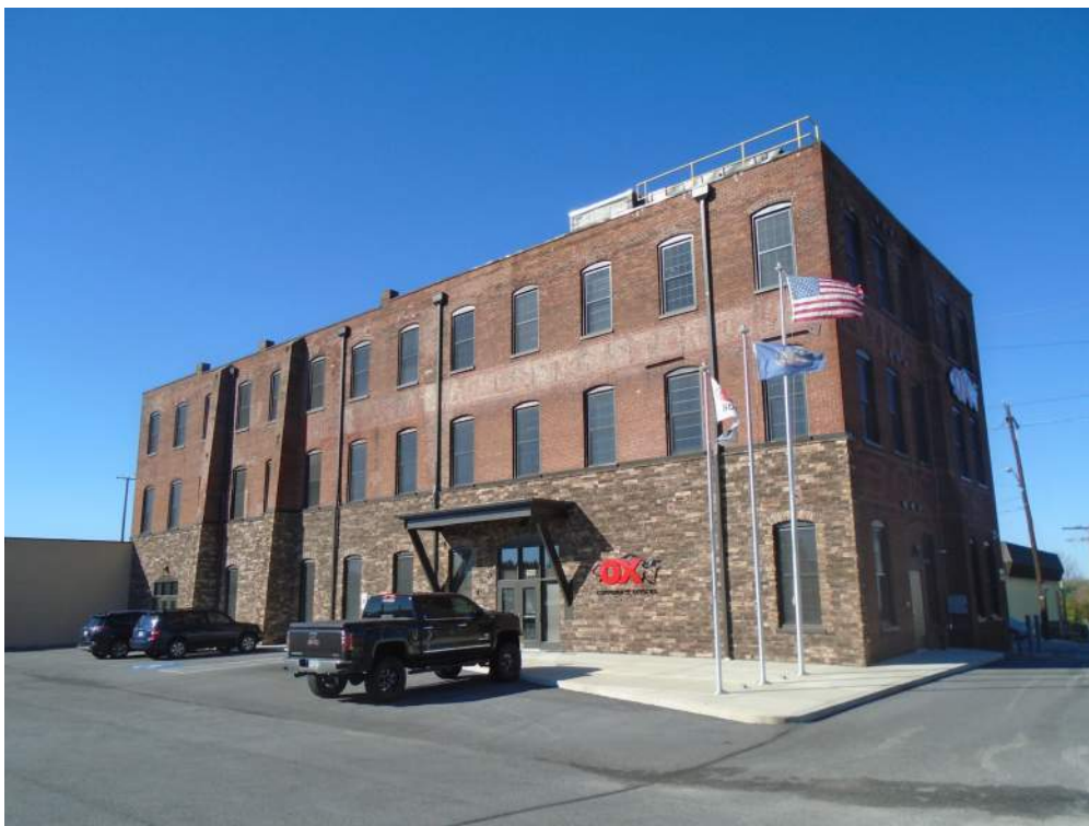
Photograph 7: The south elevation of the 1892 factory, showing the replacement windows and new stone veneer at the ground floor (2017). Looking northwest.
