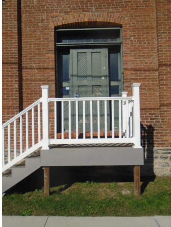
Photograph 3: Detail view of the c. 1904 factory facade, showing the historic, wood door and replacement steps and balusters. Looking north.
