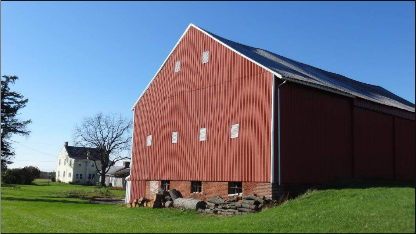
Photograph 25 – Facade (east elevation) and side (south elevation) of the Divine Chapel barn; looking northwest.
