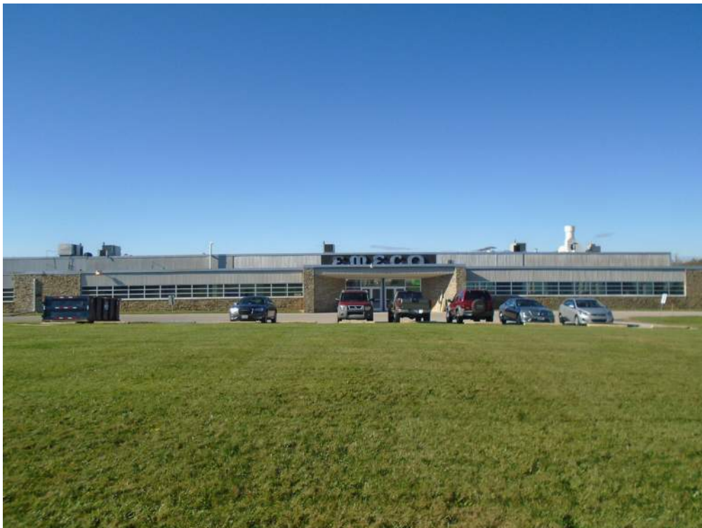
Photograph 4: The original 1950s building, showing the one-and-one-half factory and Emeco signage behind the office facade. Looking northwest.
