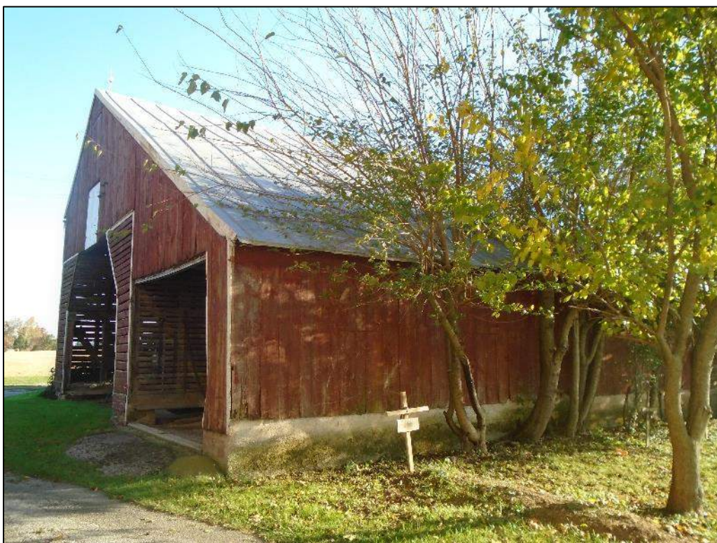
Photograph 26 – Front (west elevation) and side (south elevation) of the drive thru corn crib; looking northeast.
