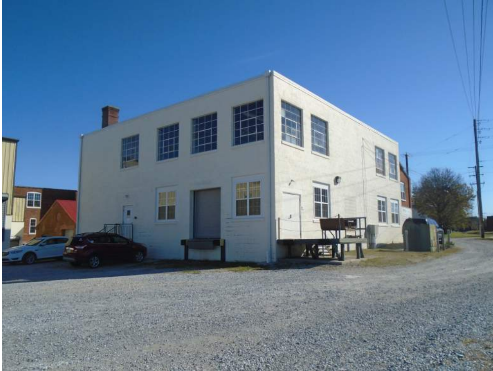
Photograph 13: The mid-twentieth century, CMU addition, showing the north and west elevations. Looking southeast.
