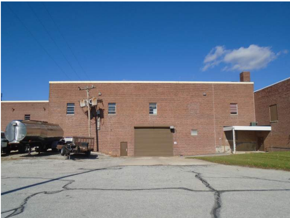
Photograph 20: The south elevation of the 1967 addition, showing the west elevation of the 1971 addition to the far right. Looking north.
