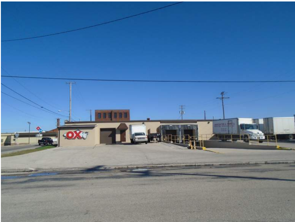
Photograph 12: West elevation of the c. 1935 addition. Looking east.
