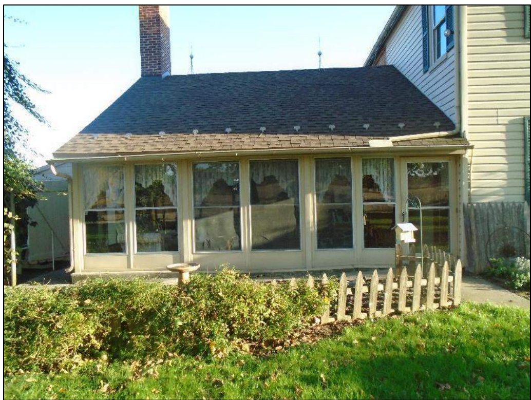
Photograph 8 – Side (south elevation) of the summer kitchen; looking north.
