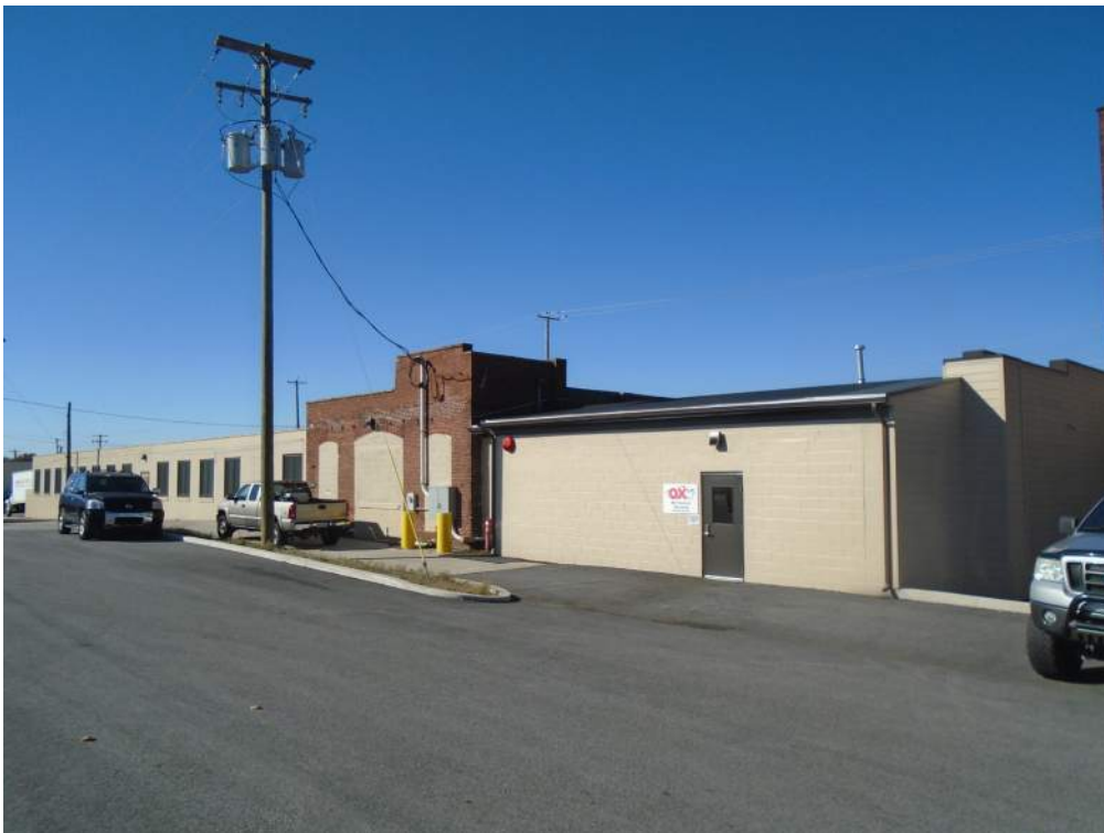
Photograph 14: South elevation of buildings "E" and "G" (c. 1935, CMU addition), which is on either side of building "E" (2017). Looking northwest.
