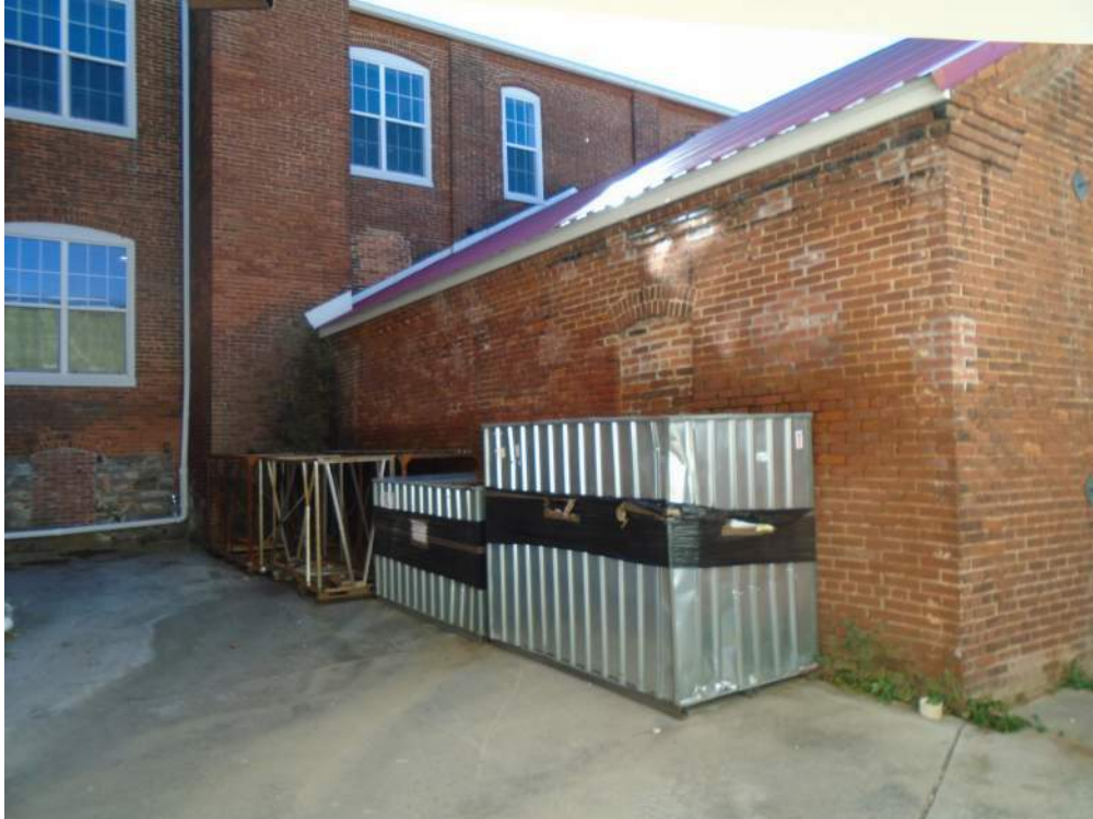
Photograph 9: The engine room ell, showing the east elevation and the first bay of the main building's south elevation at left. Looking southwest.
