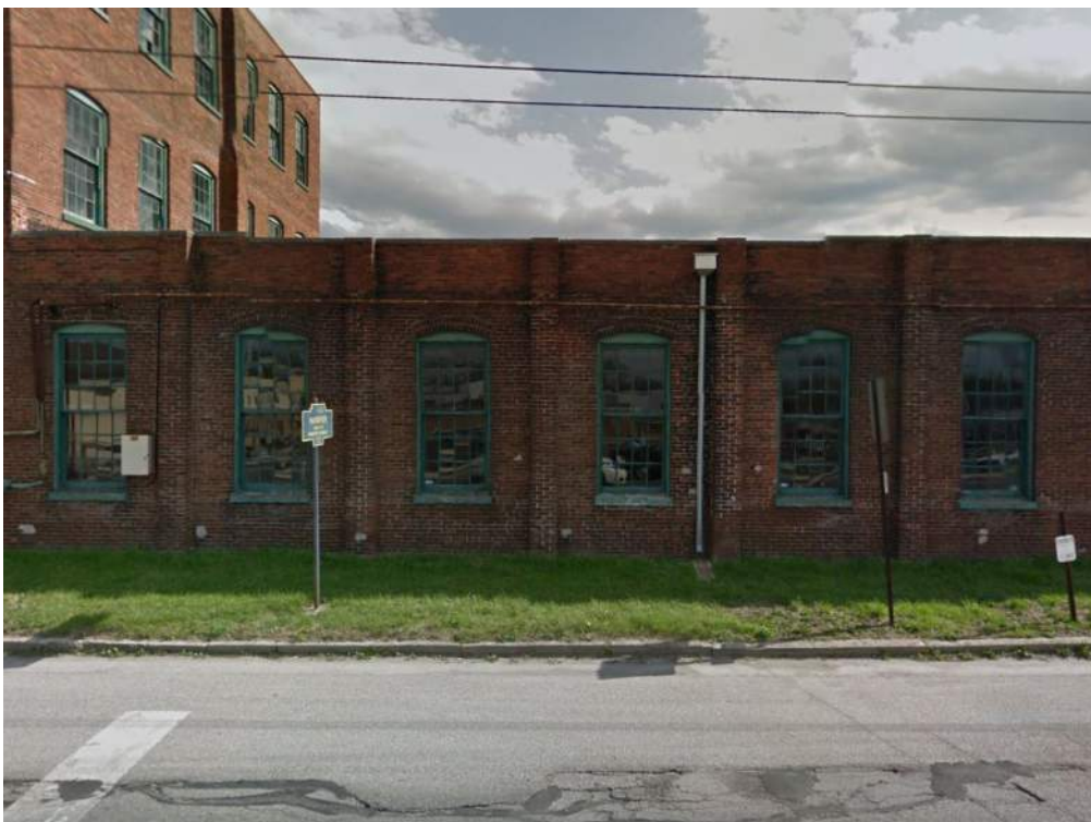
Photograph 6: Facade (north) of the c. 1910 addition, showing the historic, twelve-over-twelve, wood windows still in place, c. 2012 (Google Streetview). Looking south.
