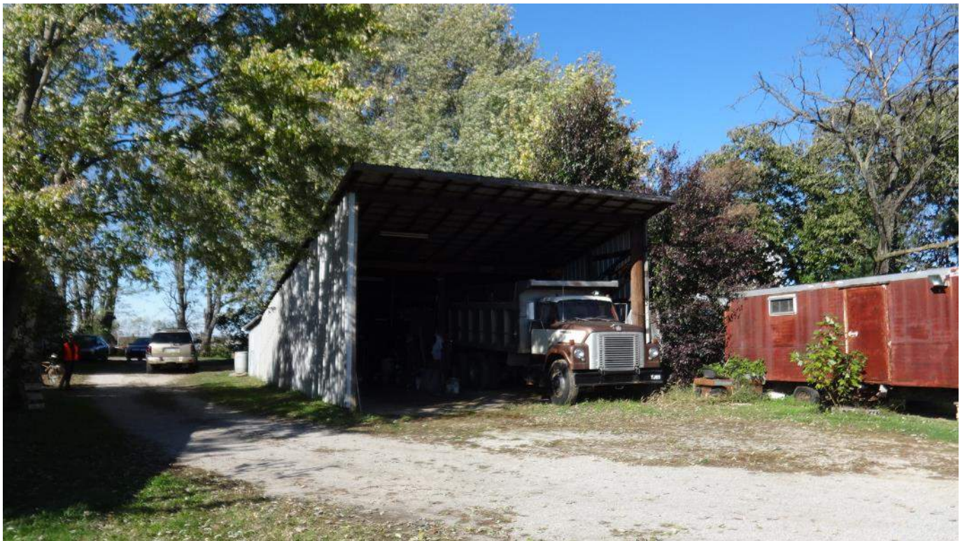
Photograph 8 – Southeast and southwest elevatons of the Poist Farm garage; looking north.
