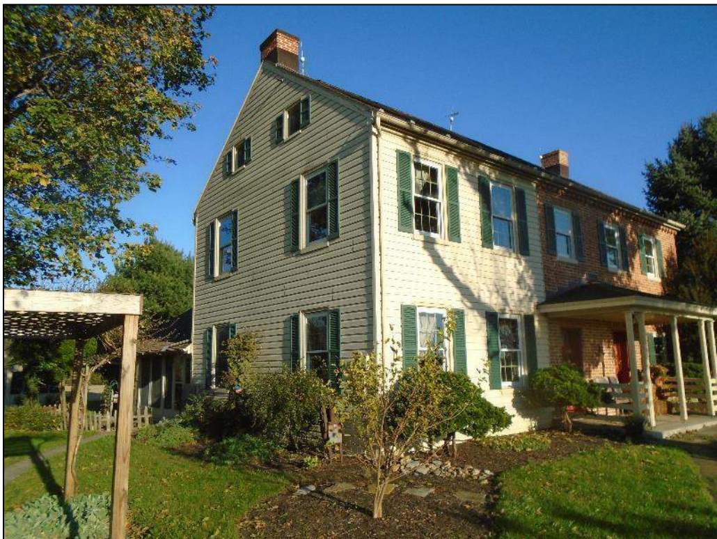
Photograph 5 – Façade (east elevation) and side (south elevation) of the dwelling; looking north.
