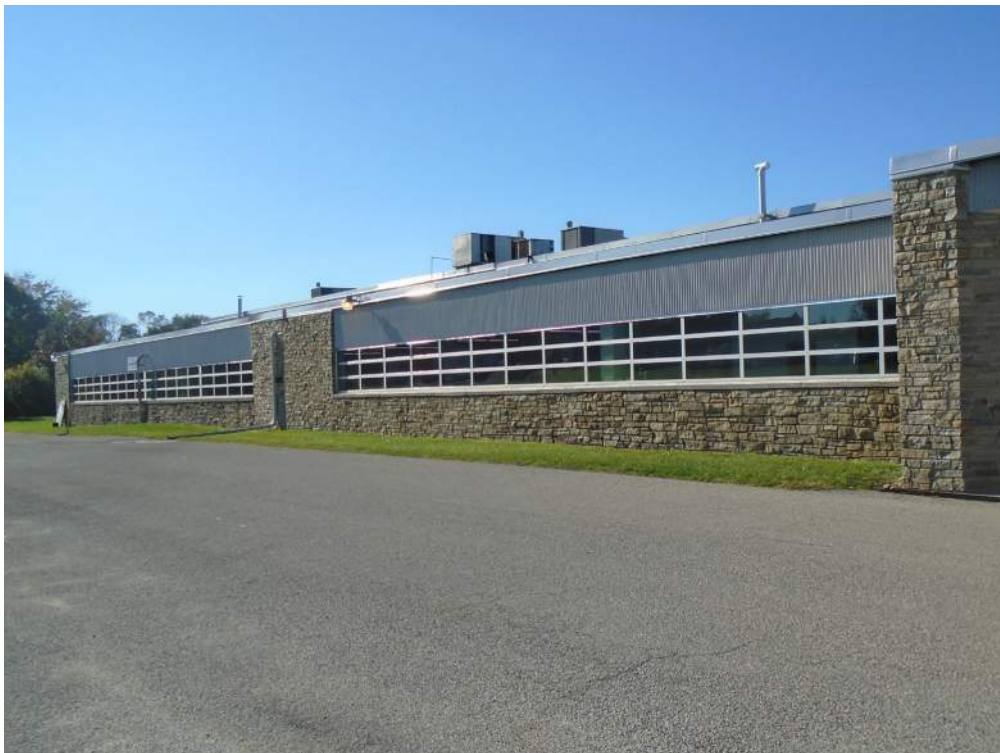
Photograph 2: The 1968 addition and 1950s building (left to right), showing the replacement ribbon windows and corrugated metal infill above. Looking southwest.
