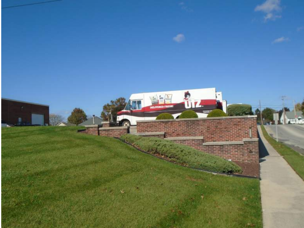
Photograph 29: The retaining wall on the east side of the complex north, located northwest of the 1971 addition. Looking north.
