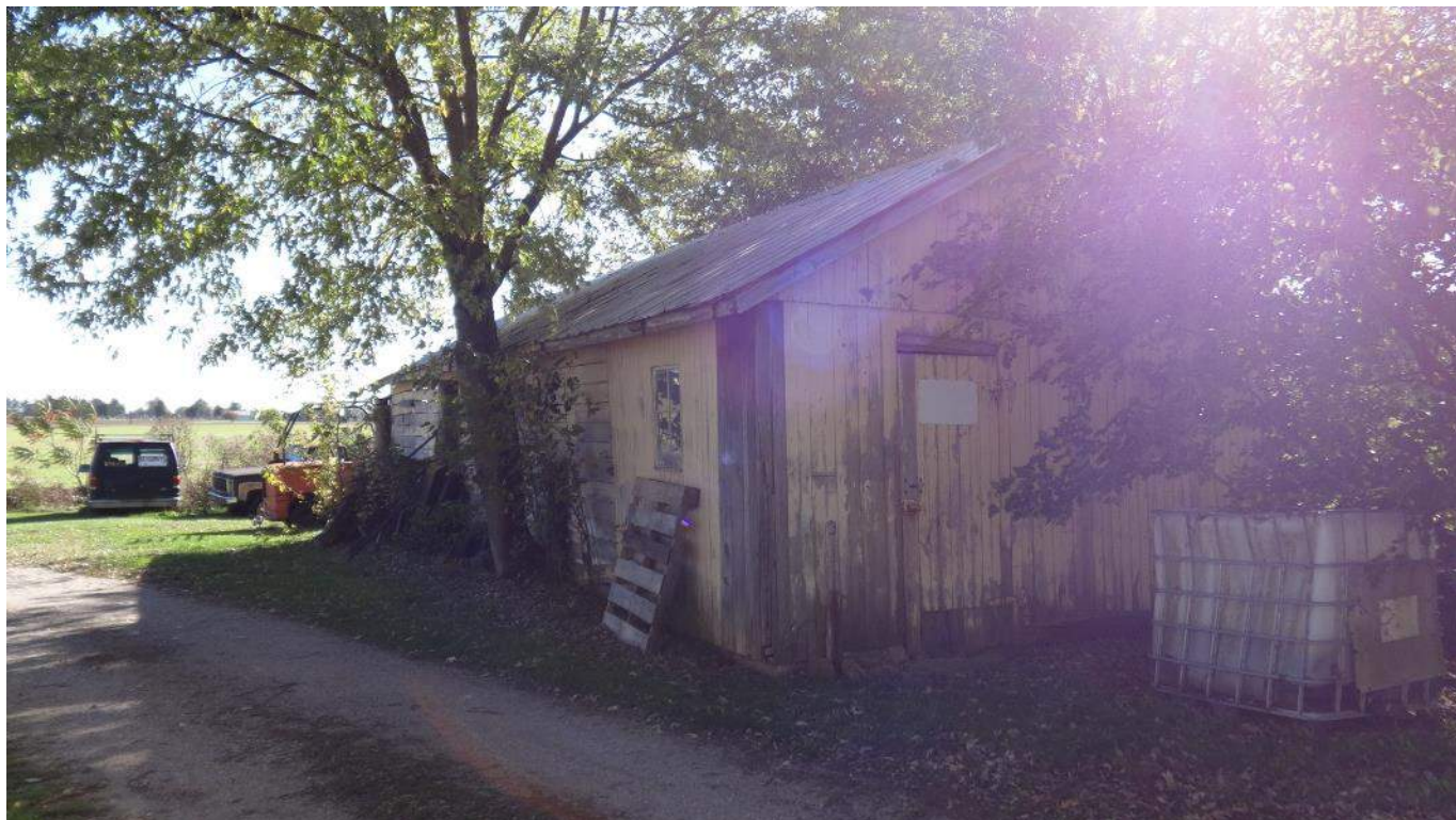
Photograph 13 – North and east elevations of the Poist Farm hog house; looking south.
