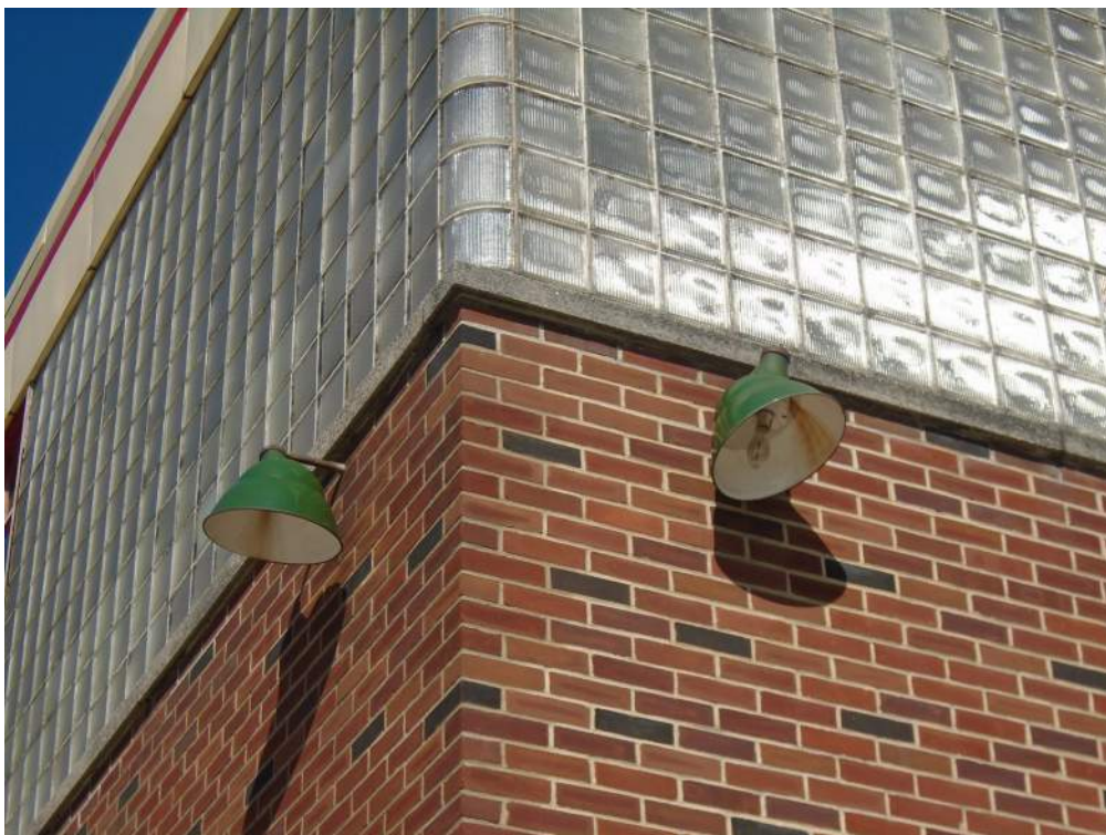
Photograph 16: Detail view of the southwest corner, showing the curved glass block and original light fixtures. Looking northeast.
