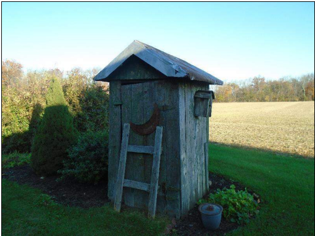
Photograph 13 – Front (south elevation) and side (east elevation) of the privy; looking northwest.
