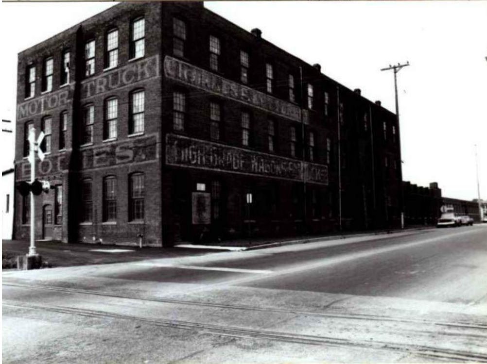
Photograph 1: The 1892 factory, showing the east and north elevations (1984). Looking southwest.
