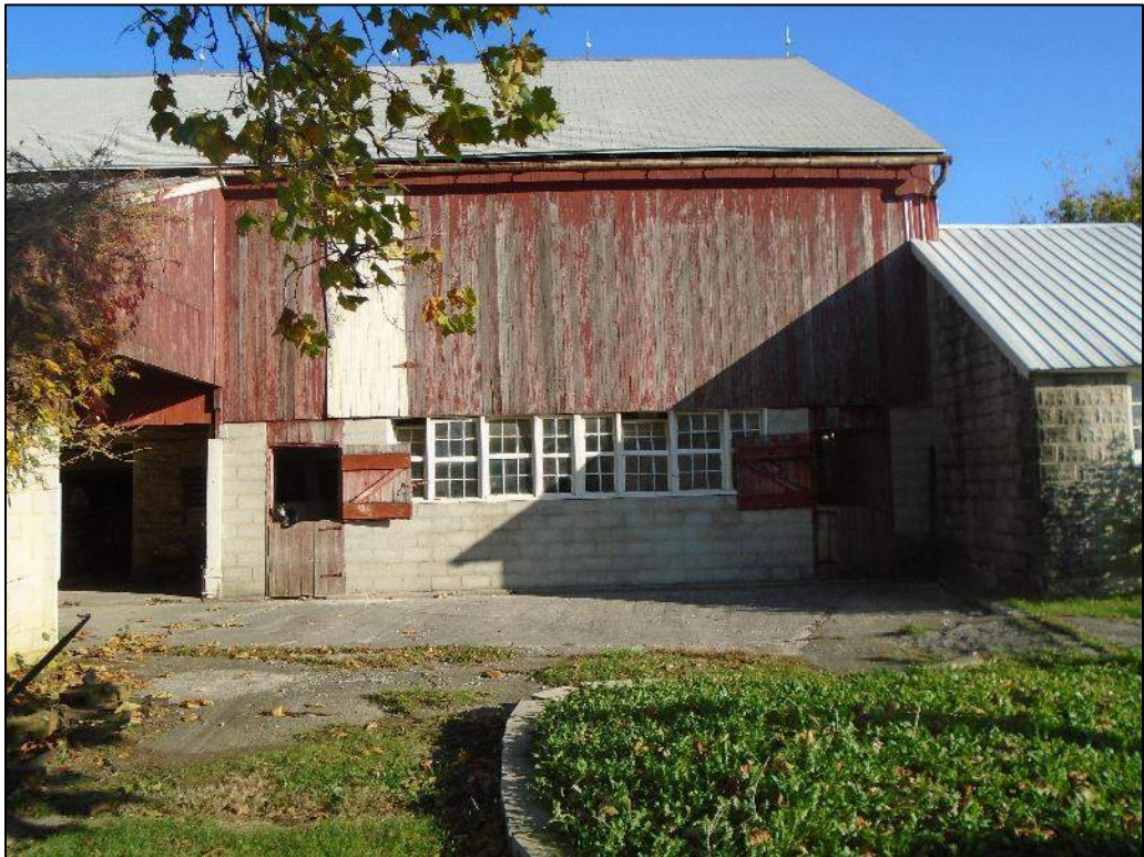
Photograph 22 – Rear (south elevation) of the barn with milk house and addition; looking north.
