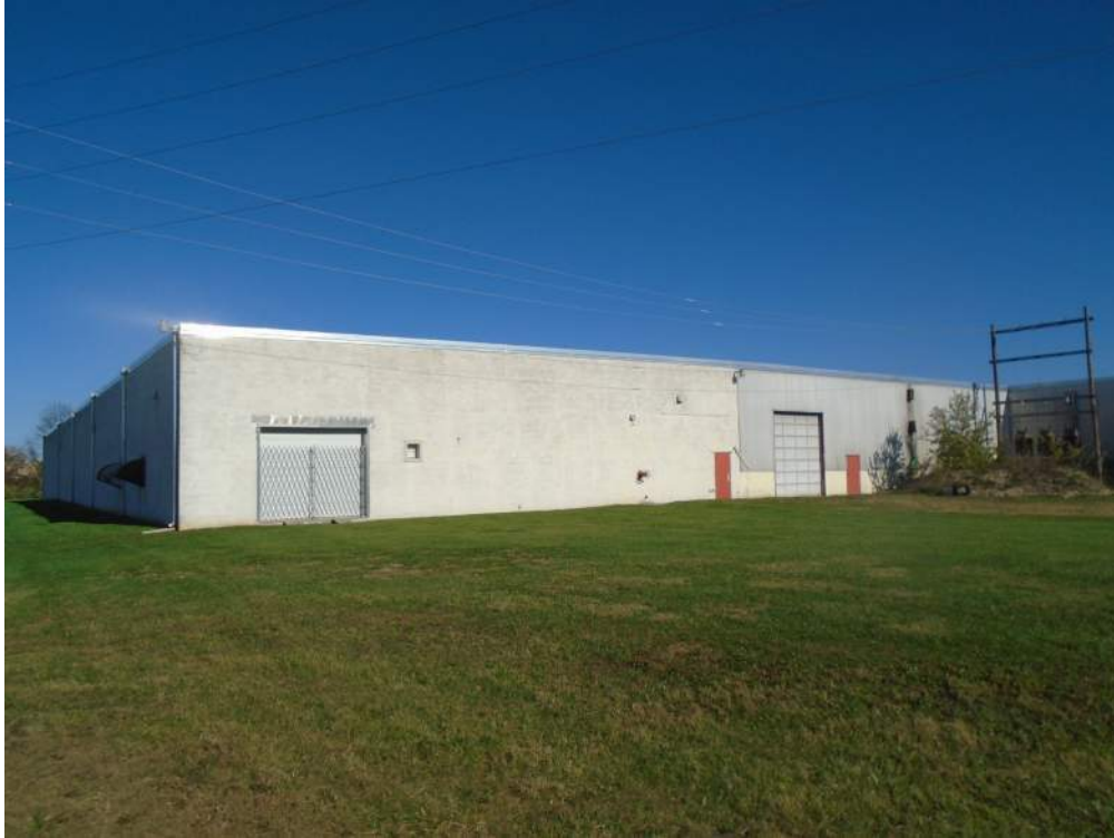
Photograph 13: The post-1971 and late 1960s additions (left to right), showing the southwest elevation. Looking east.
