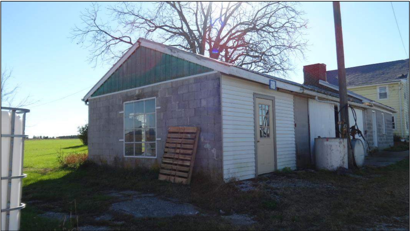
Photograph 22 – Rear (east elevation) and side (north elevation) of the Divine Chapel milkhouse; looking southwest.
