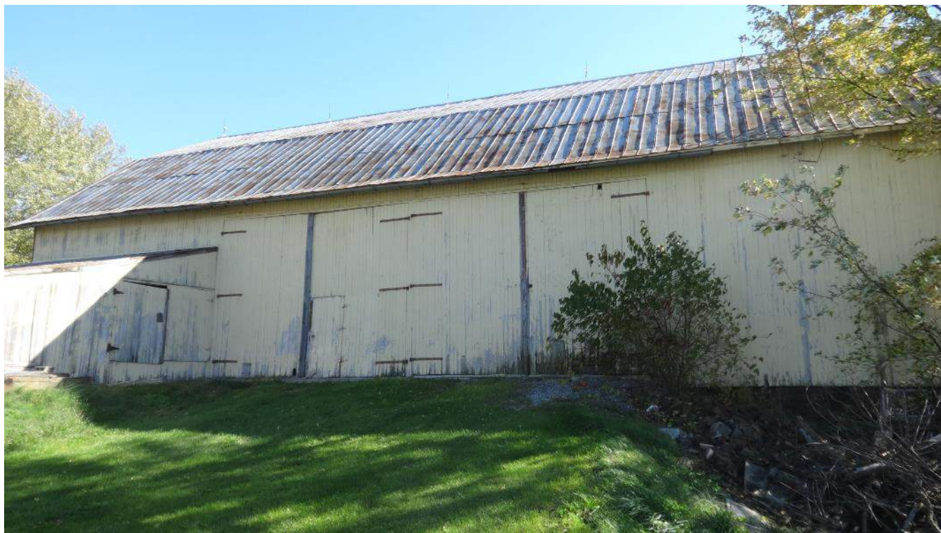
Photograph 10 – Northwest elevaton of the Poist Farm barn; looking southeast.
