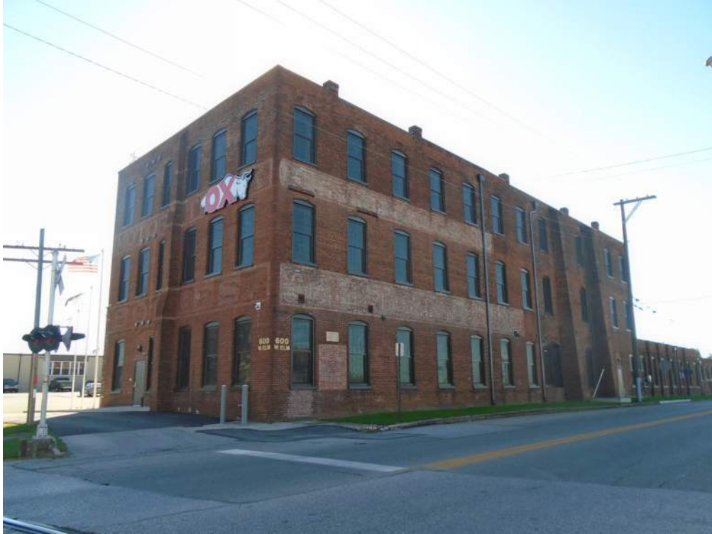
Photograph 9: Facade (north) and east elevation of the 1892 factory, as well as the c. 1910 addition to the far right (2017). Looking southwest.
