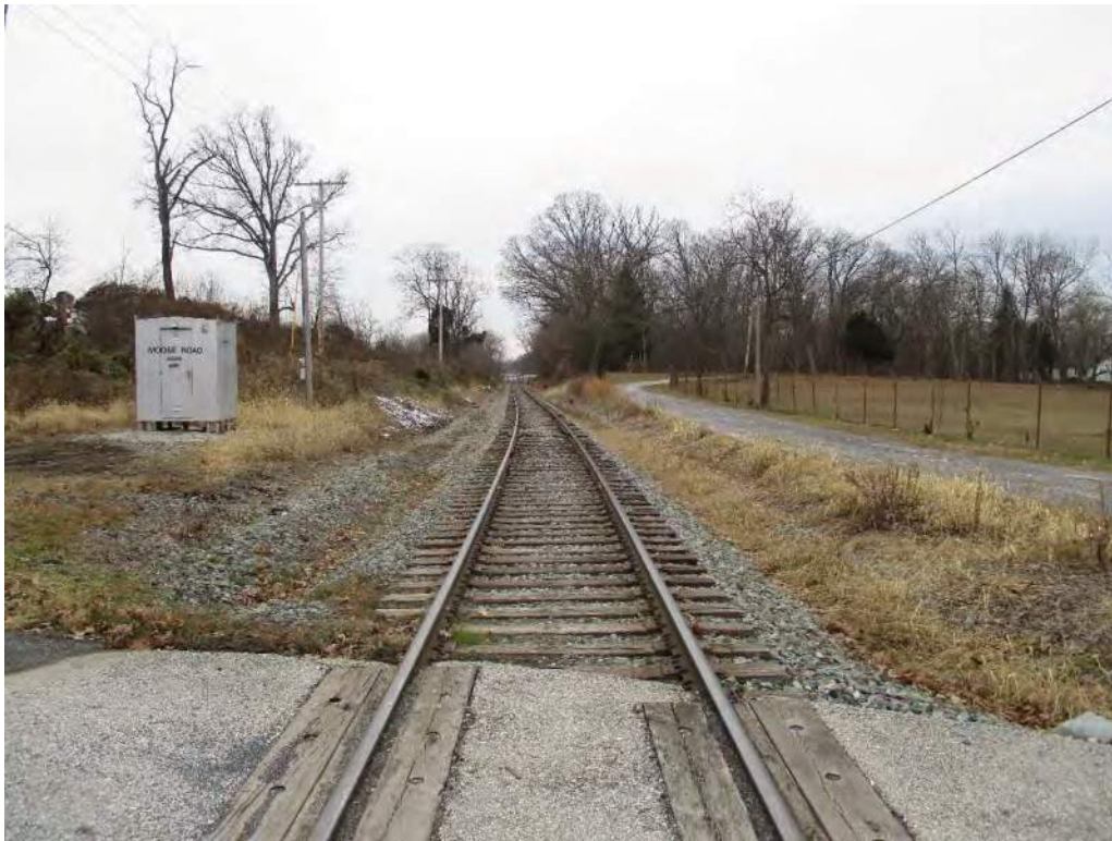
Photograph 21: View of the former Gettysburg Railroad alignment, approaching Gettysburg, from the Moose Road crossing looking west.
