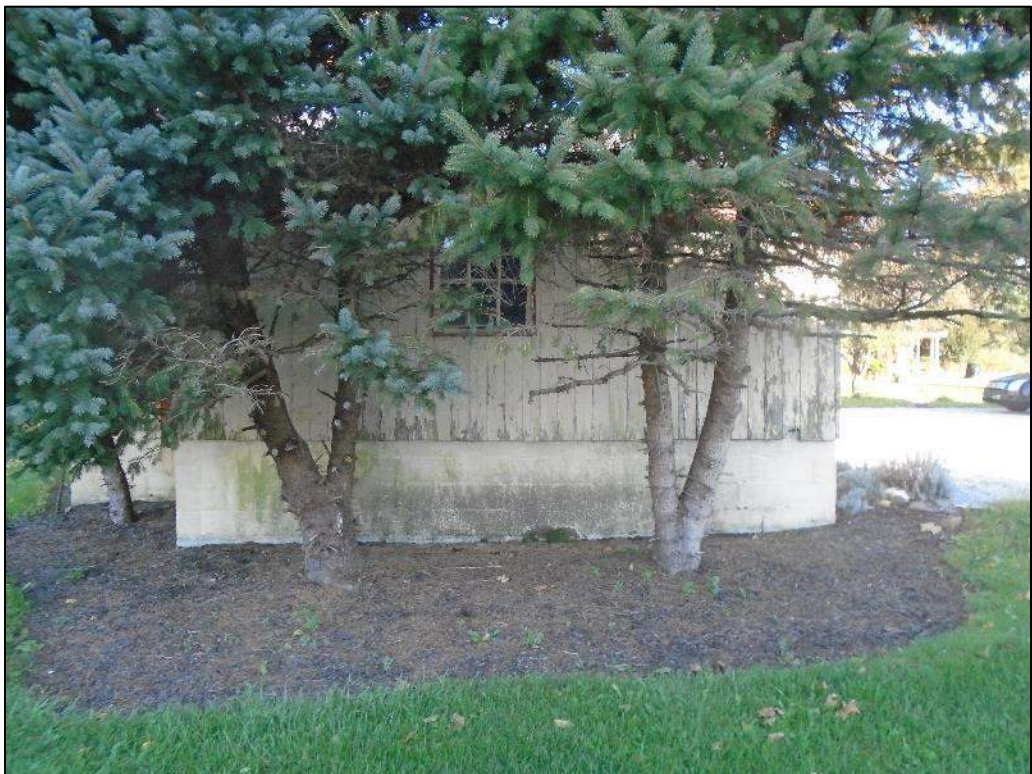
Photograph 16 – Rear (southwest elevation) of the machine shed addition; looking northeast.
