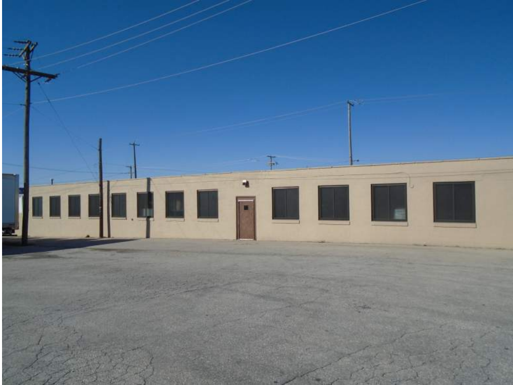
Photograph 13: South elevation of the c. 1935 addition. Looking northwest.
