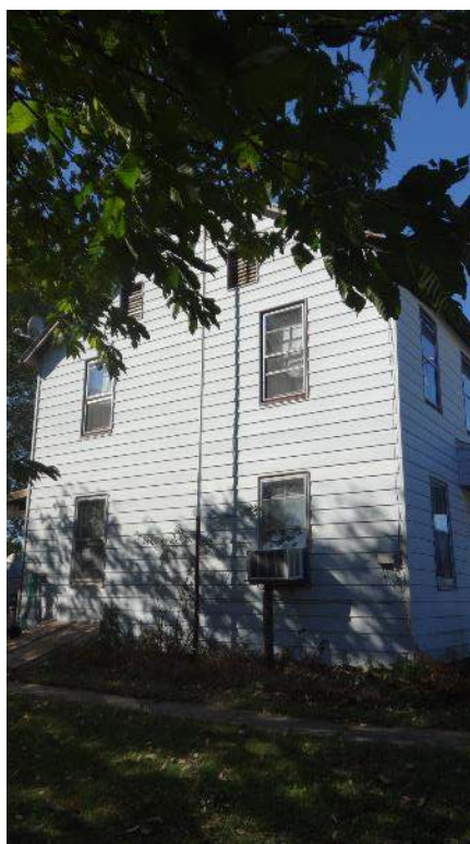
Photograph 2 – Side (southeast elevation) of the Poist Farm dwelling; looking northwest.
