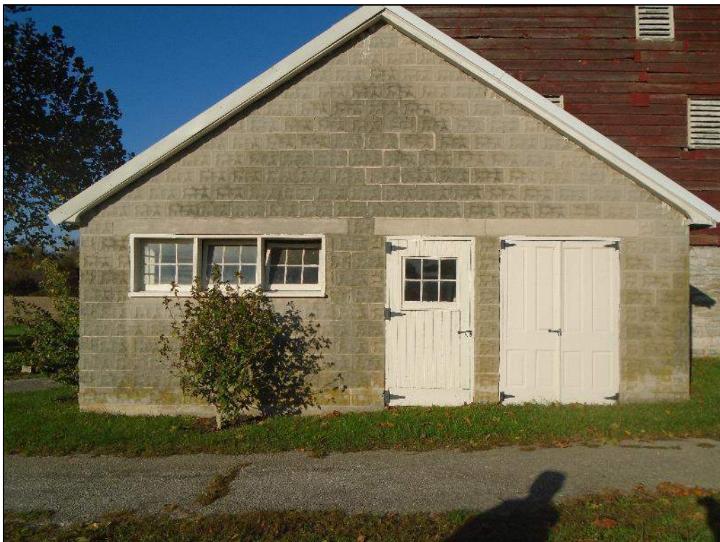
Photograph 23 – Front (east elevation) of the milk house addition; looking west.
