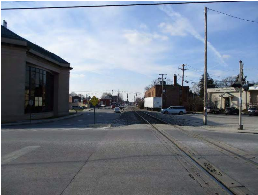
Photograph 3: View of the former Gettysburg Railroad alignment, in Hanover at 3 rd Street and North Railroad Street, looking west.
