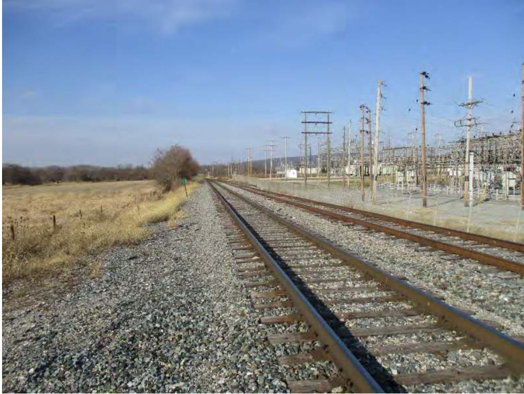
Photograph 7: View of the former Gettysburg Railroad alignment, leaving Hanover, at the Radio Road crossing, looking north-northwest.
