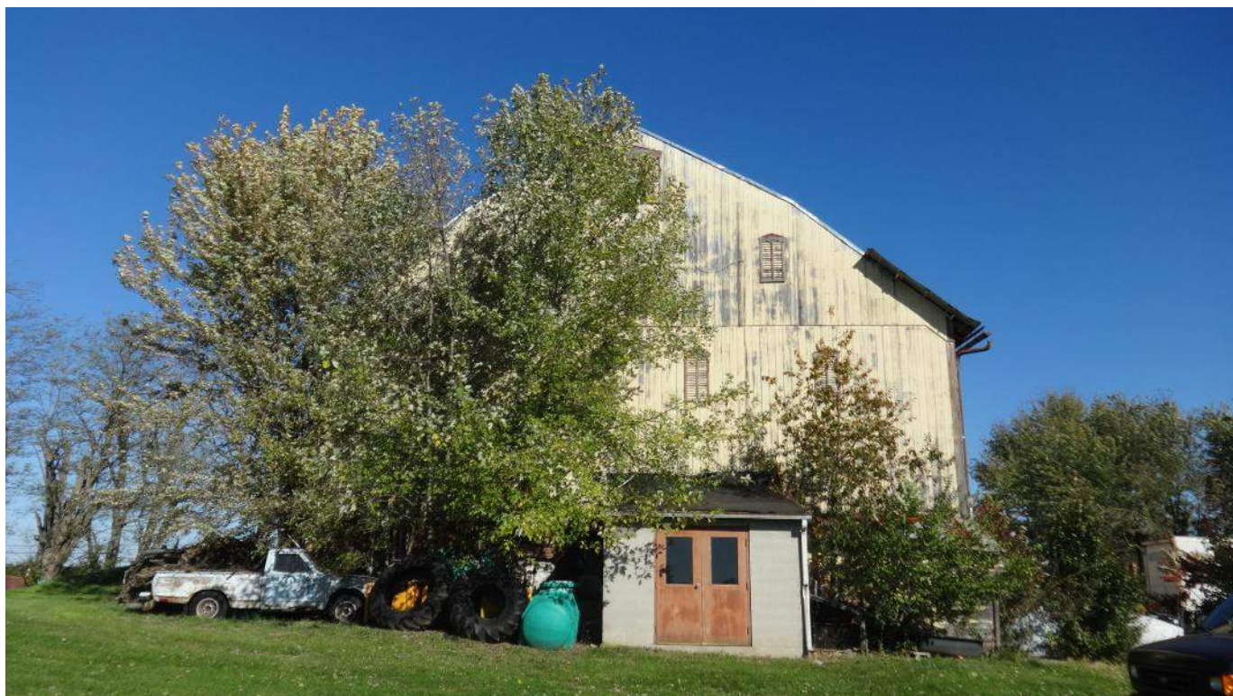
Photograph 11 – Southwest elevation of the Poist Farm barn; looking northeast.
