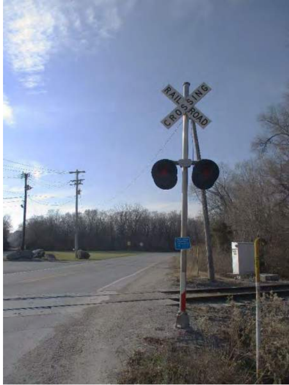
Photograph 9: View of the grade crossing signal, outside of Hanover, at the Hanover Street crossing, looking west.
