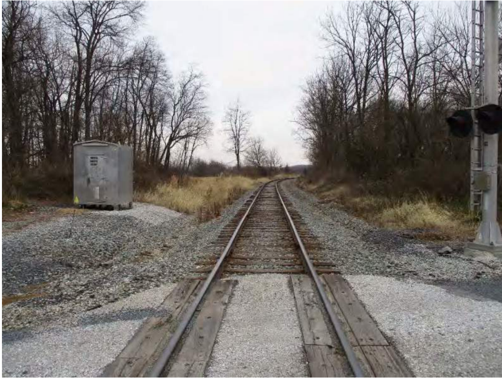
Photograph 23: View of the former Gettysburg Railroad alignment, approaching Gettysburg, from the Smith Road crossing looking east.
