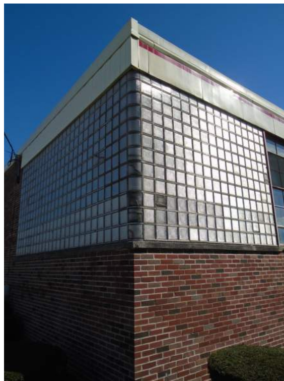
Photograph 12: Detail view of the curved glass block glazing and metal fascia at the northwest corner. Looking southeast.
