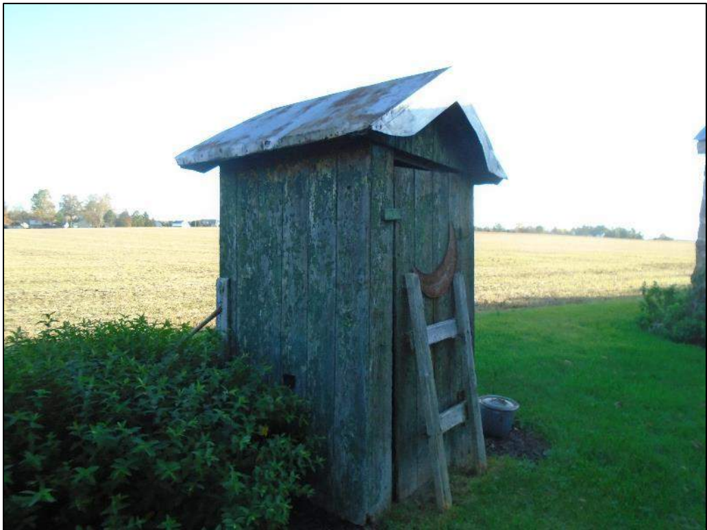
Photograph 11 – Front (south elevation) and side (west elevation) of the privy; looking northeast.
