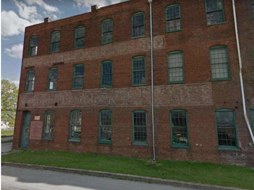
Photograph 5: Facade (north) of the 1892 factory, showing the historic, twelve-over-twelve, wood windows still in place, c. 2012 (Google Streetview). Looking southeast.
