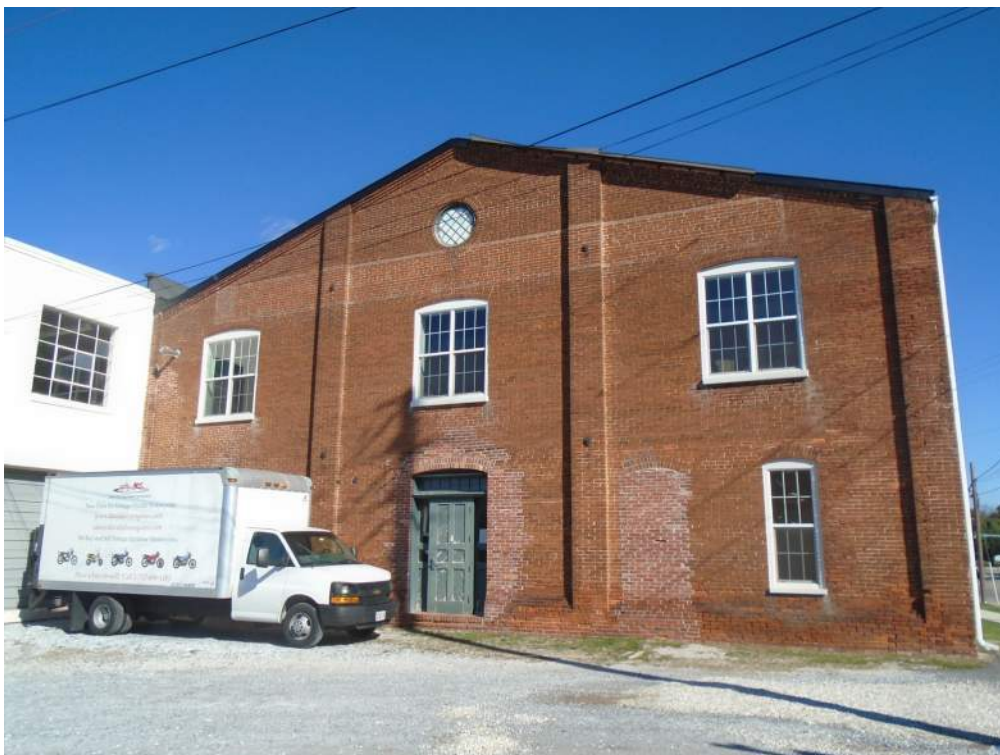
Photograph 6: The c. 1904 factory, showing the west elevation as well as the mid-twentieth century addition to the north. Looking east.
