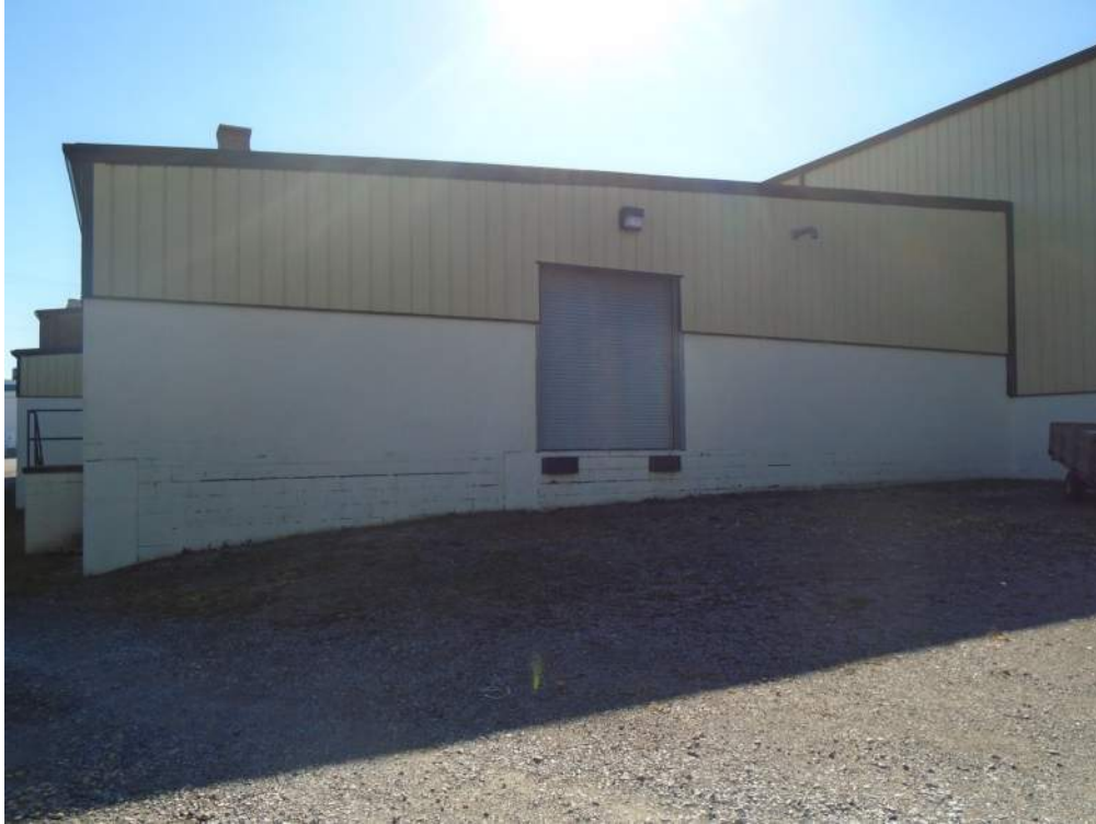
Photograph 17: The post-1971, storage addition, showing the north elevation of the central section. Looking south.
