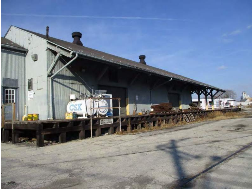
Photograph 31: View of the Western Maryland Freight Depot (Key No. 073592), looking north.
