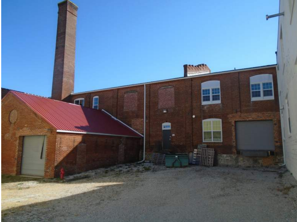
Photograph 5: The c. 1904 factory, showing the north elevation as well as the engine room ell and chimney. Looking southeast.
