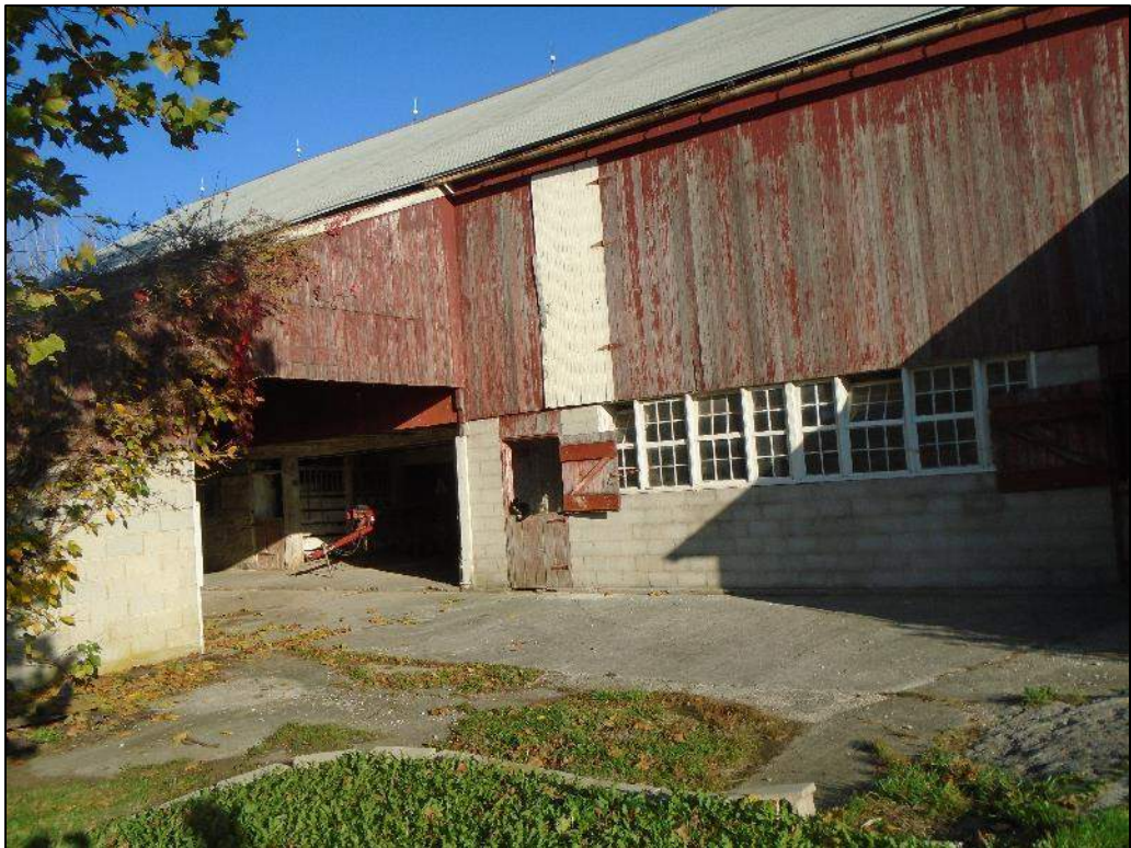
Photograph 21 – Rear (south elevation) of the barn and side (east elevation) of the addition; looking northwest.
