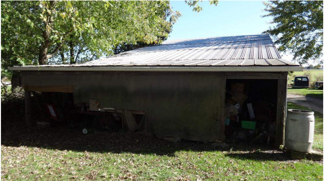
Photograph 7 – Northwest elevaton of the original Poist Farm chicken coop; looking southeast.
