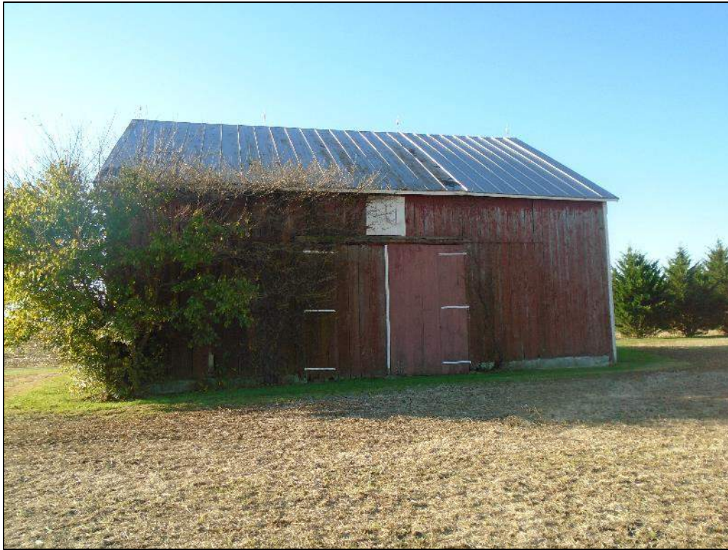
Photograph 33 – Rear (north elevation) of the hay drying shed; looking south.
