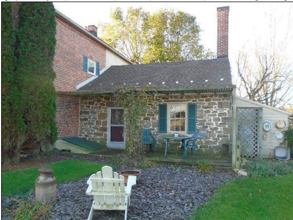
Photograph 6 – Side (north elevation) of the summer kitchen and rear (west elevation) of the dwelling; looking south.
