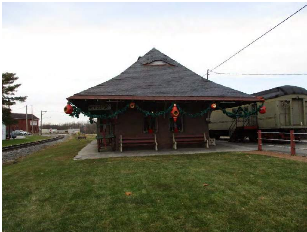
Photograph 34: View of the New Oxford Passenger Station, looking northwest.
