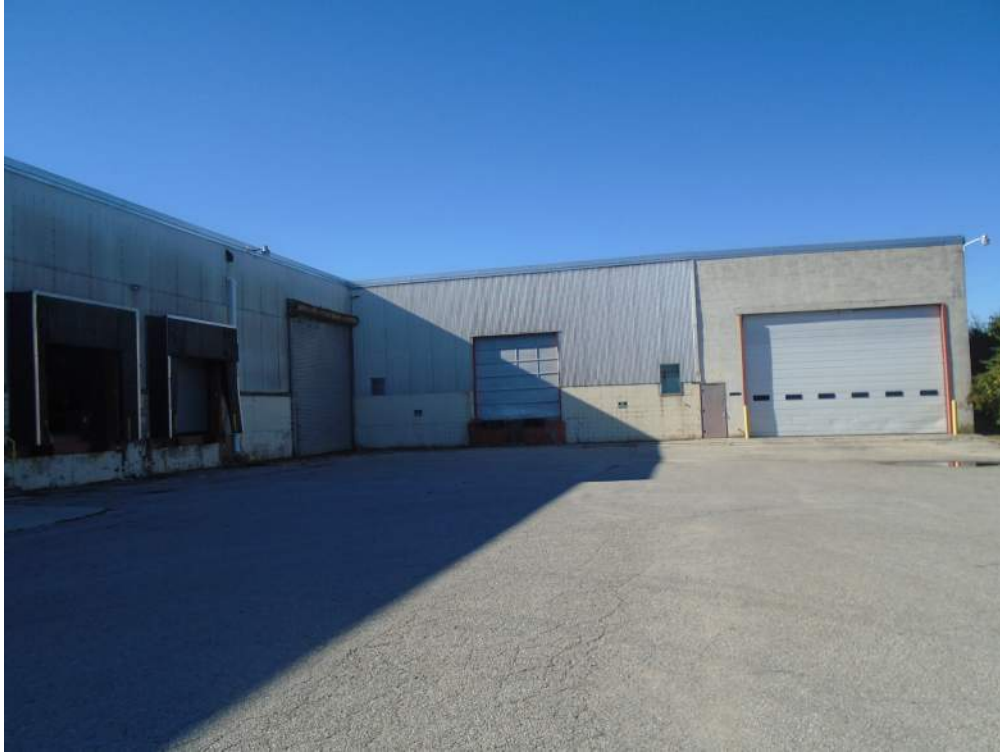
Photograph 9: The additions at the northeast corner of the 1950s factory, showing the late 1960s and post-1971 additions (left to right). Looking north.
