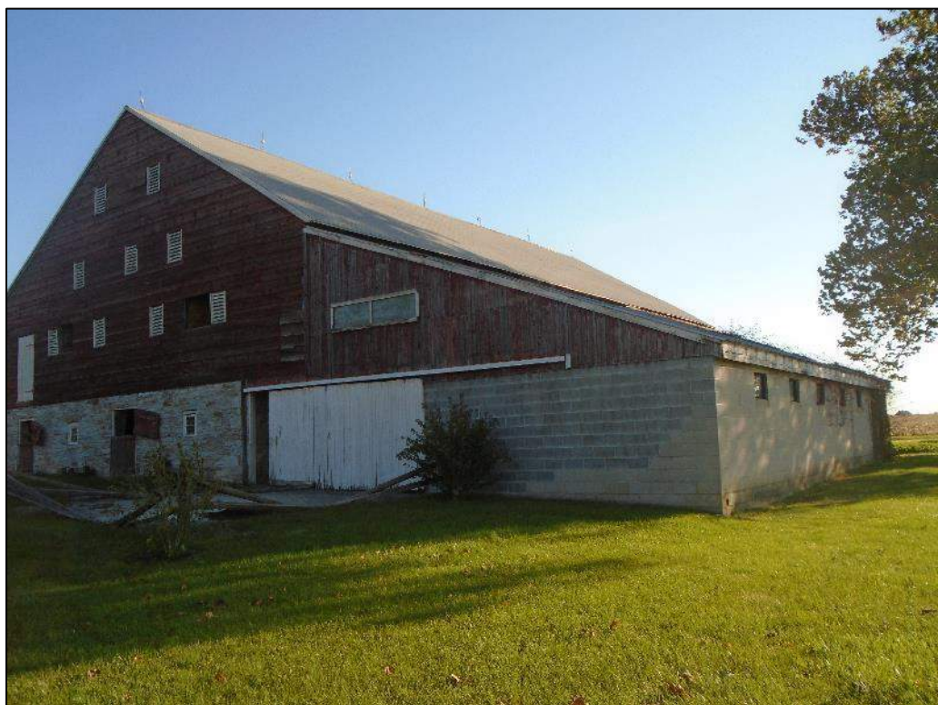
Photograph 20 – Side (west elevation) of the barn and addition and rear (south elevation) of the addition; looking east.
