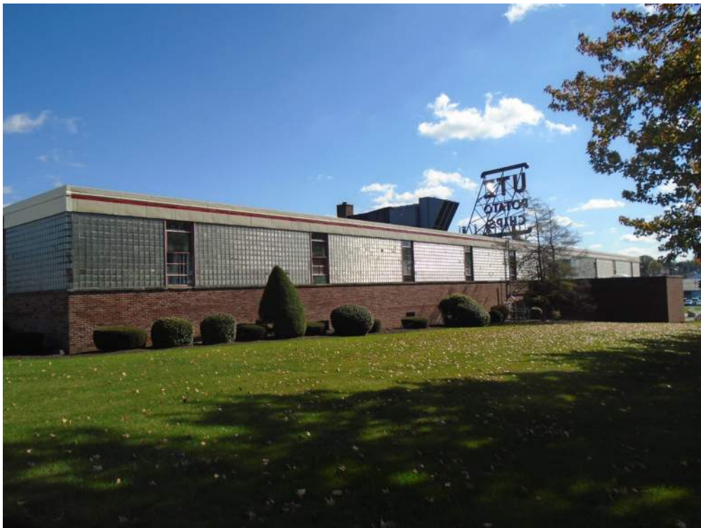
Photograph 14: The west elevation of the c. 1949 building, showing the band of glass block glazing with interspersed steel windows. Looking southeast.
