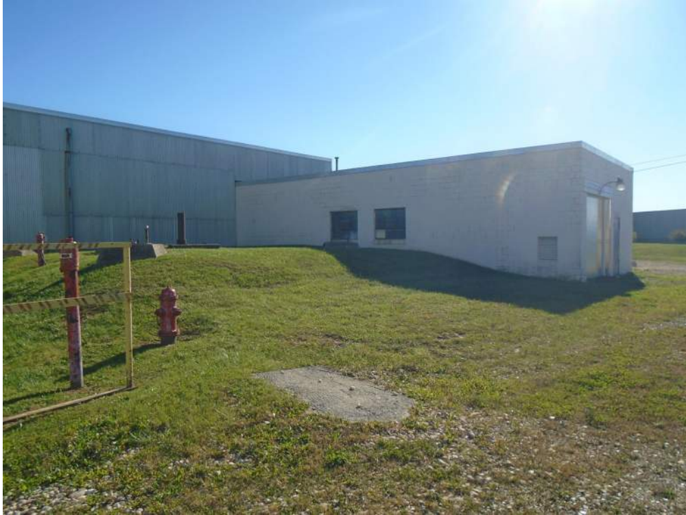
Photograph 15: Detail view of the CMU structure attached to the 1968 addition. Looking southwest.
