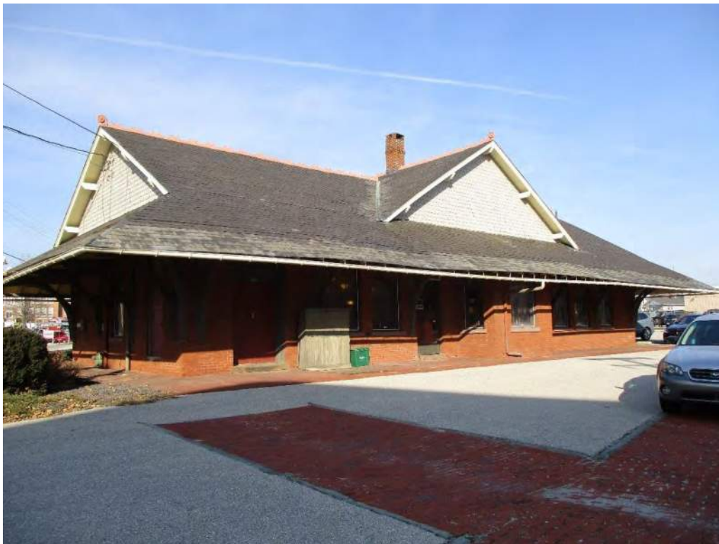
Photograph 28: View of the rear of the Hanover (Union) Passenger Station (facing the tracks of the former Gettysburg Railroad), looking south.
