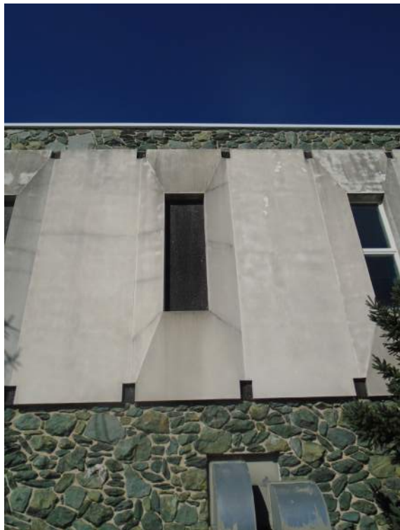
Photograph 23: Detail view of the pyramidal concrete panels and coarse-aggregate concrete opening infill at the south elevation of the 1971 addition. Looking north.
