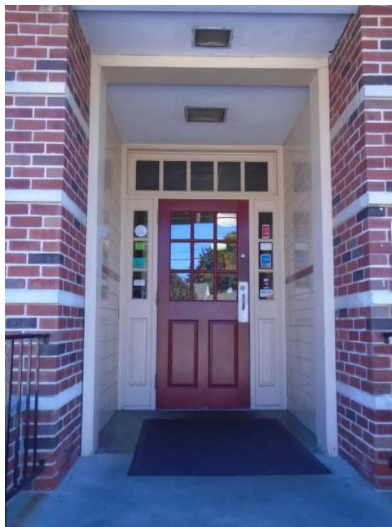
Photograph 8: View of the Factory Store entrance vestibule, showing the glazed brick and original wooden door system. Looking south.
