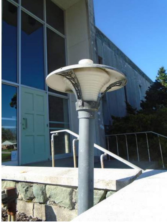
Photograph 25: Detail view of the stylized light fixture located at the north corner of the retaining wall, showing the double-height entrance behind. Looking northwest.
