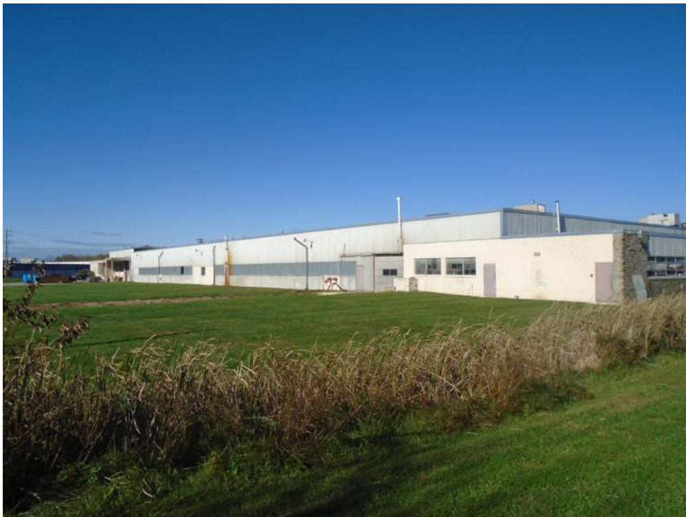
Photograph 18: The southwest elevation of the 1968 addition, showing the one-and-one-half-story factory and one-story, CMU offices (left to right).
