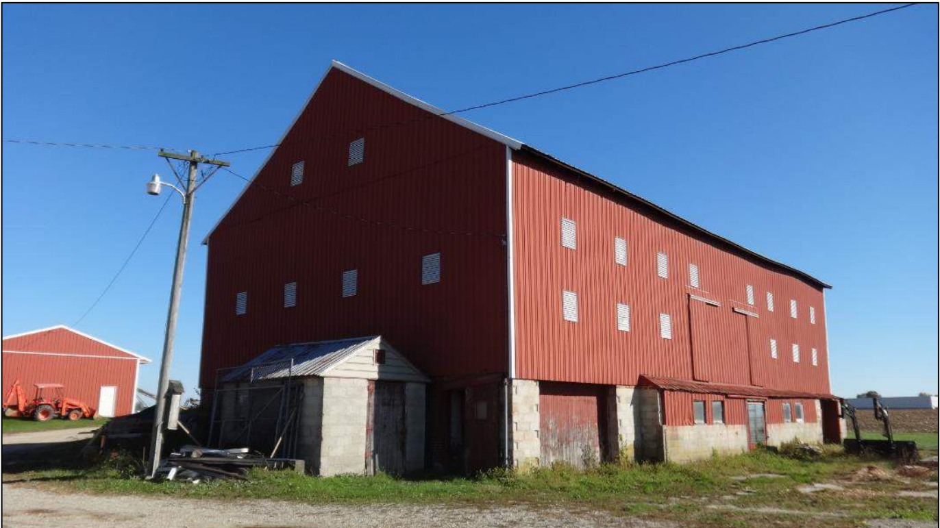
Photograph 26 – Rear (west elevation) and side (north elevation) of the Divine Chapel barn; looking southeast.
