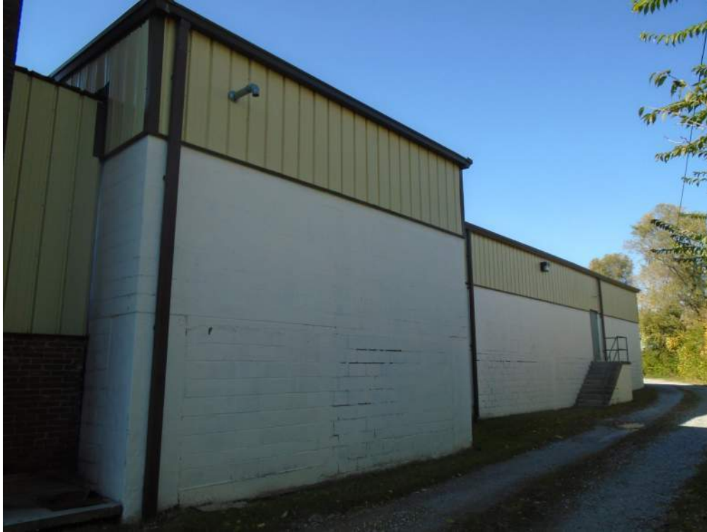
Photograph 15: The post-1971, storage addition, showing the east elevation of the southernmost section and central wing. Looking north.
