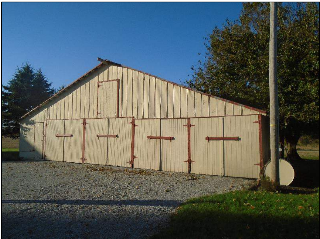
Photograph 14 – Façade (northeast elevation) of the machine shed; looking southwest.
