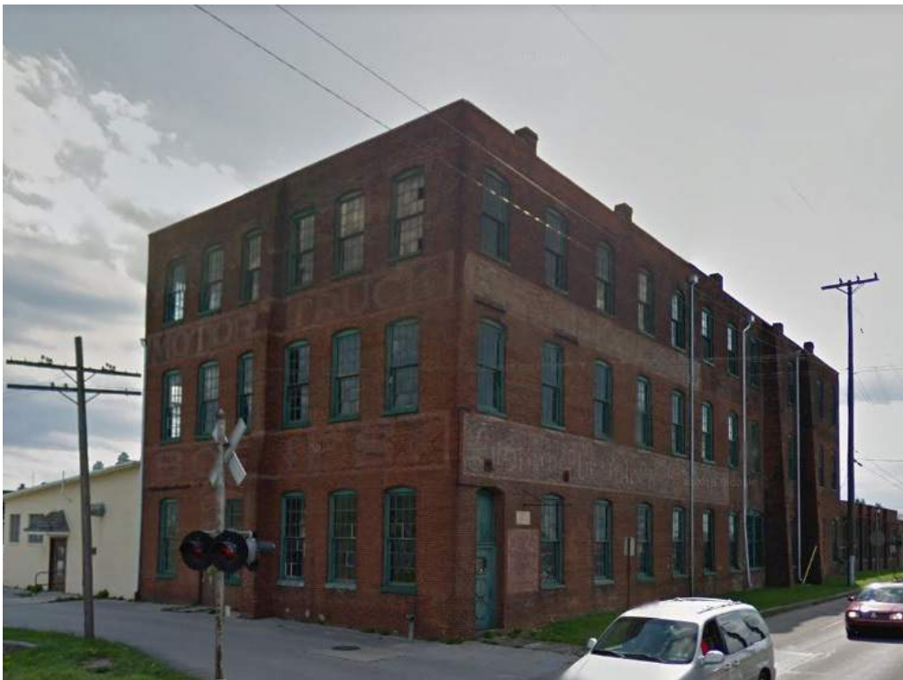
Photograph 4: The north and east elevations of the 1892 factory and east elevation of the c. 1960s addition (right to left), c. 2012 (Google Streetview). Note the historic twelve-over-twelve, wood windows in place. Looking southwest.
