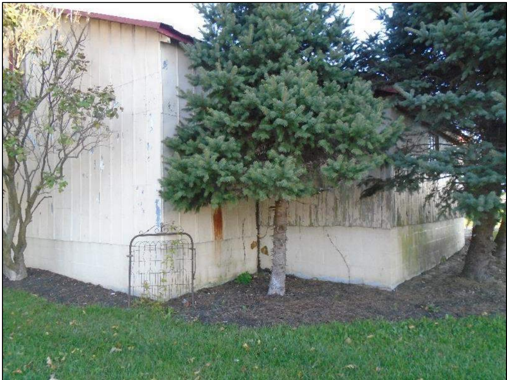
Photograph 15 – Rear (southwest elevation), side (southeast elevation) and rear (southwest elevation) of the machine shed and addition; looking north.
