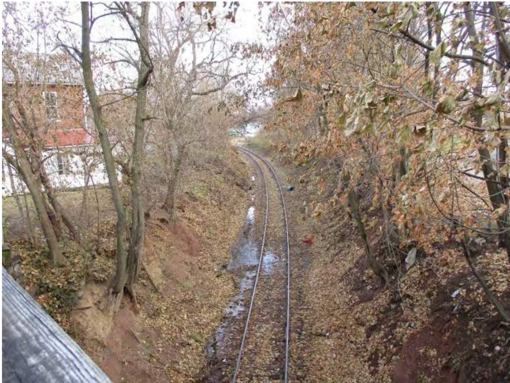
Photograph 14: View of the former Gettysburg Railroad alignment, New Oxford, at the from the High Street Bridge, looking east-southeast.
