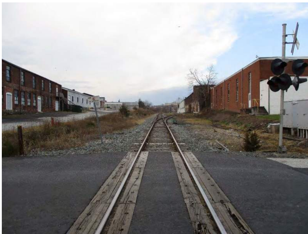
Photograph 25: View of the former Gettysburg Railroad alignment, entering Gettysburg, from the North 4 th Street crossing, looking west.
