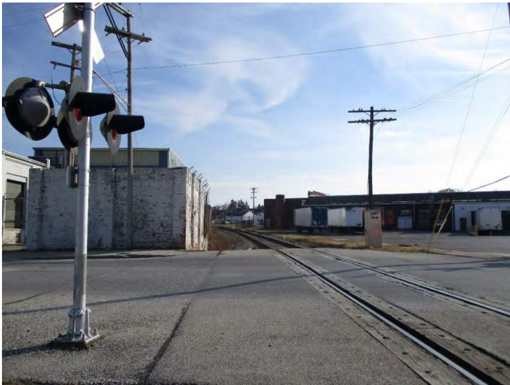
Photograph 4: View of the former Gettysburg Railroad alignment, in Hanover at the Maple Avenue crossing, looking southeast.
