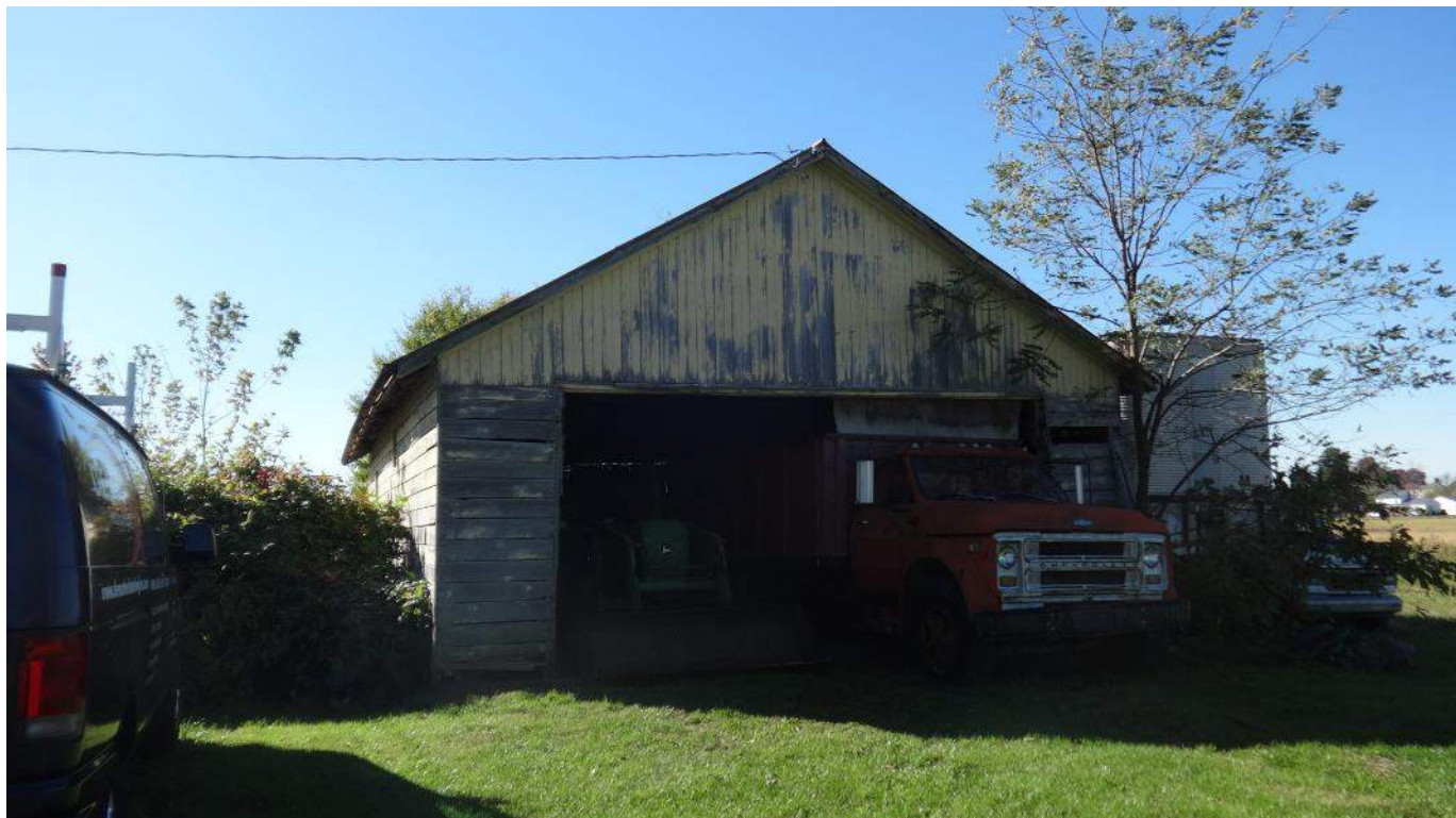
Photograph 15 – Northeast elevation of the Poist Farm corn crib; looking southwest.
