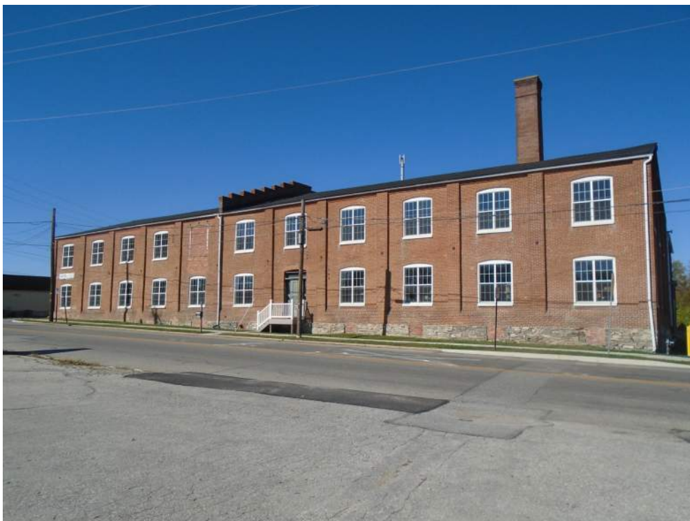
Photograph 2: The c. 1904 factory, showing the facade (south). Looking northwest.
