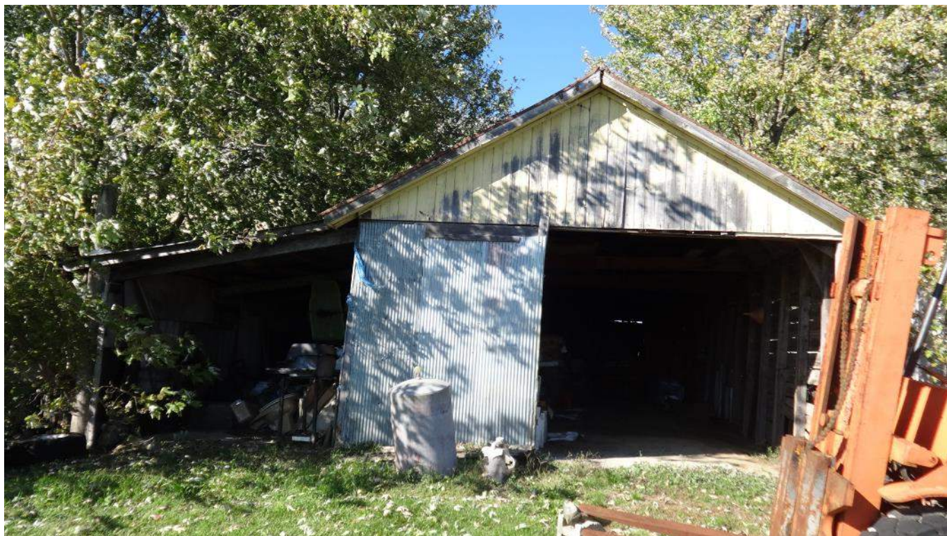
Photograph 14 – South elevation of the Poist Farm hog house; looking north.
