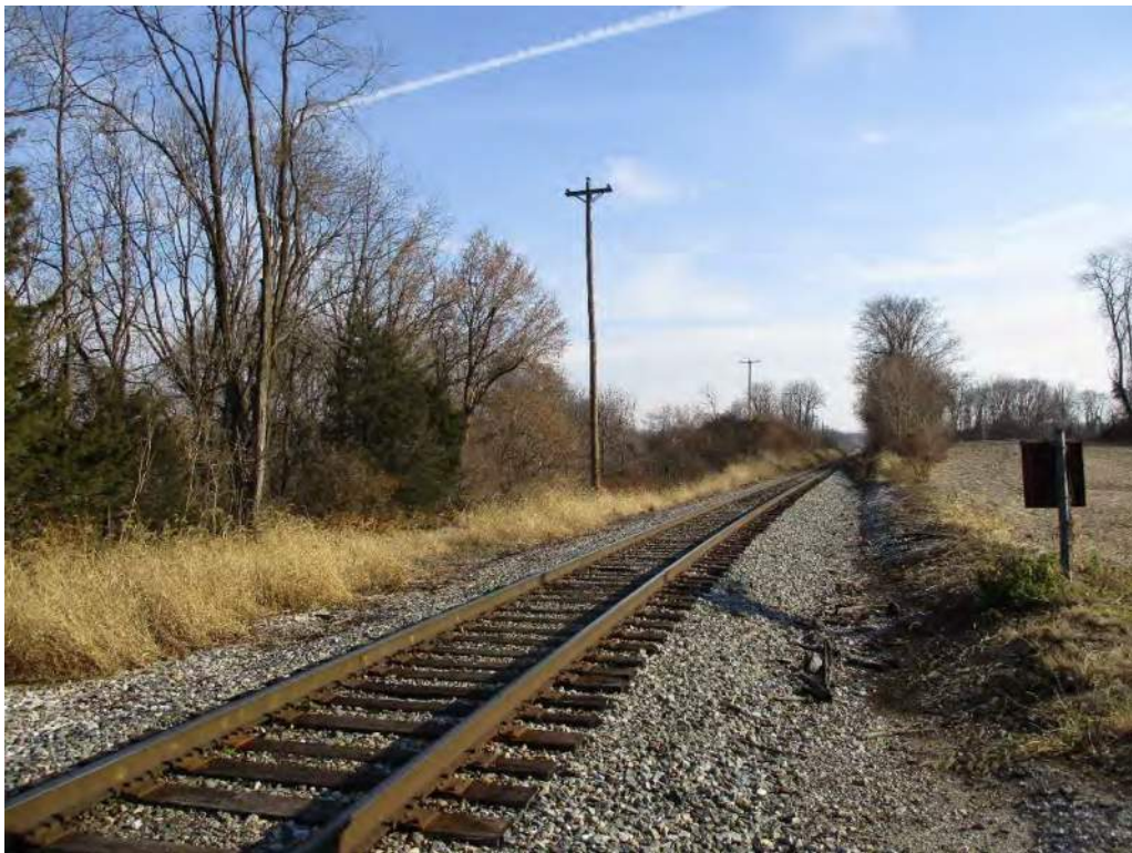
Photograph 10: View of the former Gettysburg Railroad alignment, outside of Hanover, at the Red Hill Road crossing, looking southeast.
