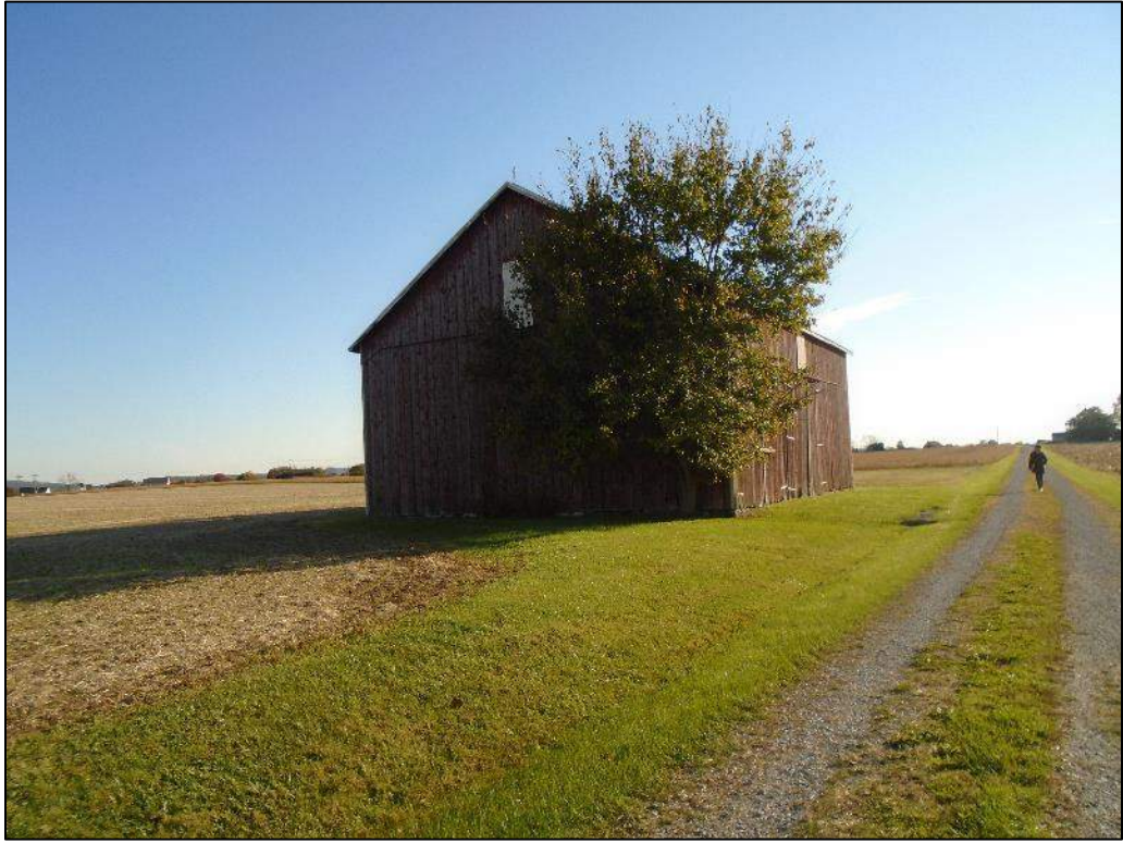
Photograph 32 – Side (west elevation) and front (south elevation) of the hay drying shed; looking east.
