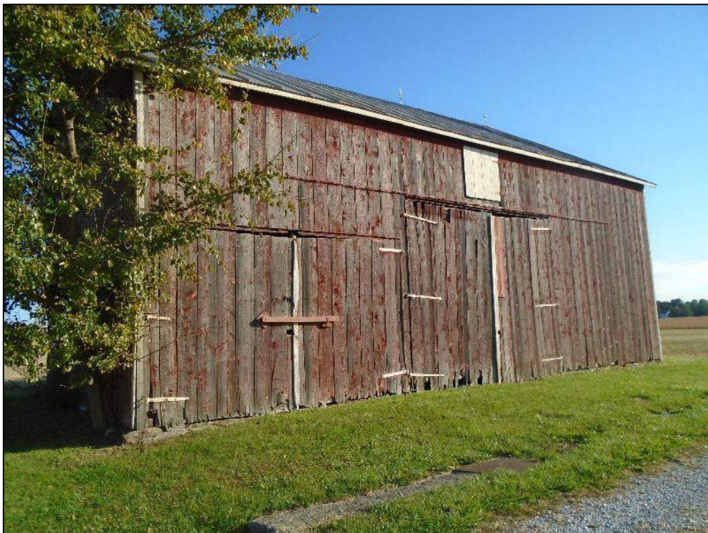
Photograph 30 – Front (south elevation) of the hay drying shed; looking northeast.
