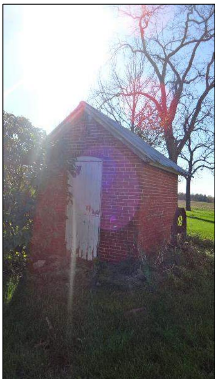
Photograph 23 – Front (east elevation) and side (north elevation) of the Divine Chapel smokehouse; looking west.
