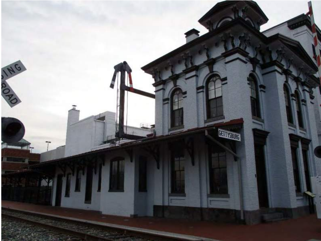
Photograph 37: View of Gettysburg Passenger Station, looking southeast.
