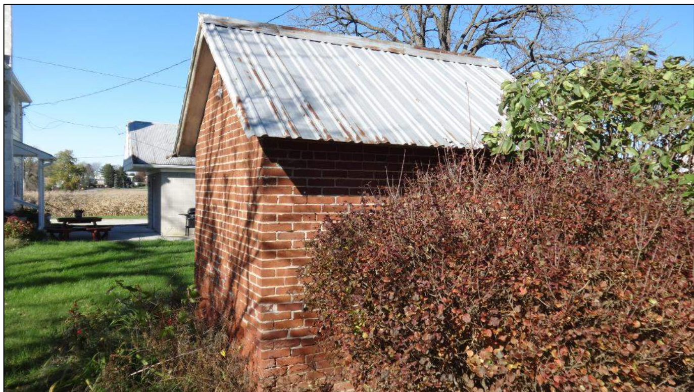
Photograph 24 – Rear (west elevation) and side (south elevation) of the Divine Chapel smokehouse; looking north.
