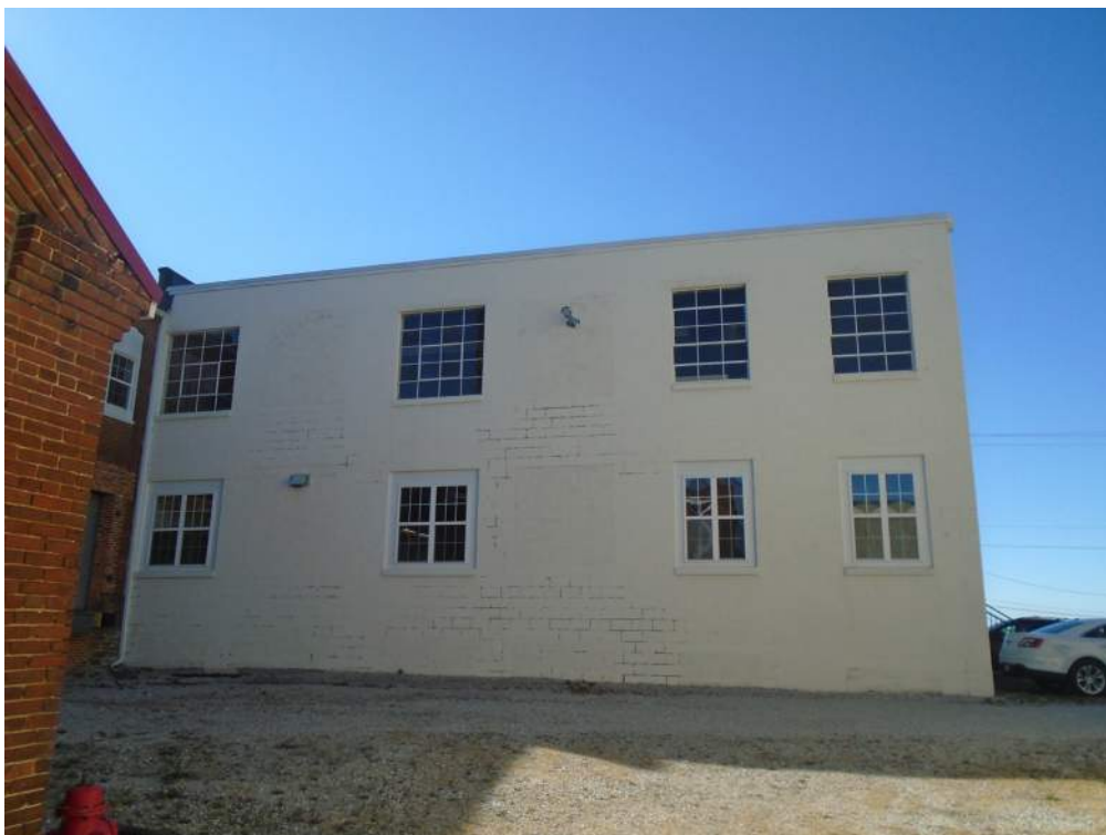
Photograph 14: The mid-twentieth century, CMU addition, showing the east elevations. Looking west.
