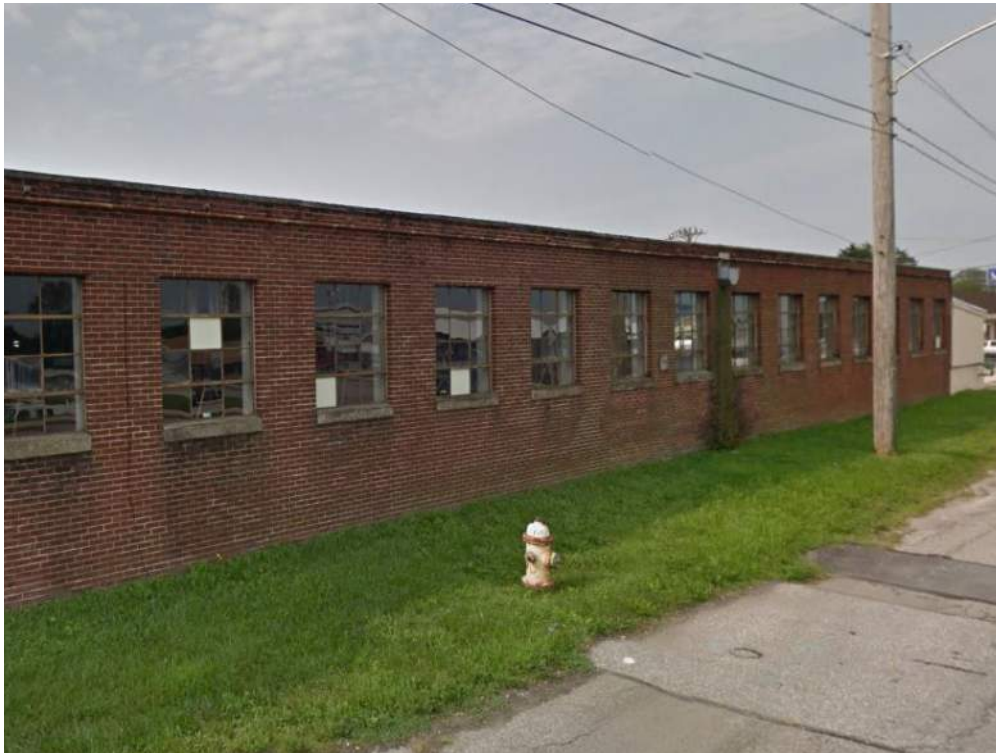
Photograph 8: North elevation of c. 1935 addition "G," showing the historic three-over-six-over-three windows still in place, c. 2012 (Google Streetview). Looking west.
