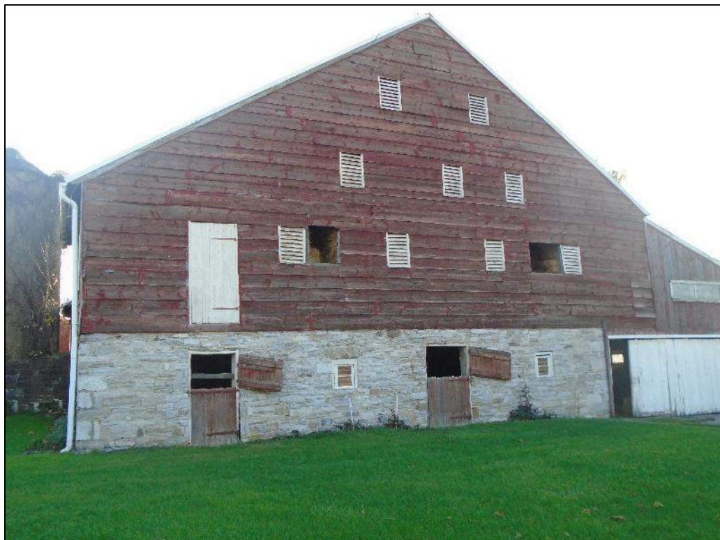
Photograph 19 – Side (west elevation) of the barn; looking east.
