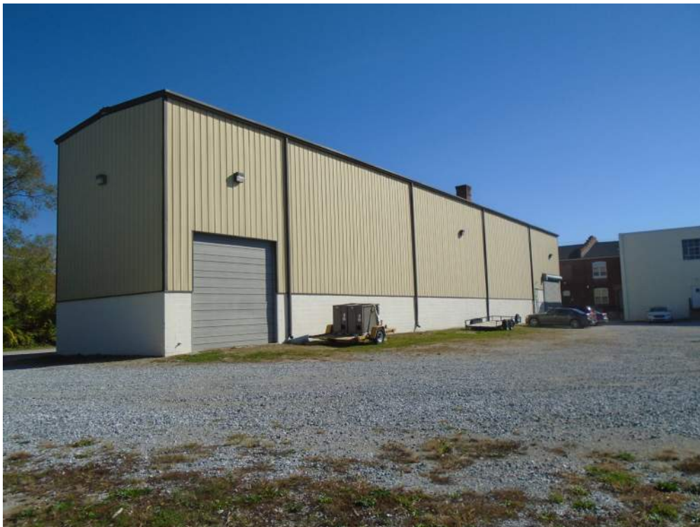
Photograph 18: The post-1971, storage addition, showing the north and west elevations of the westernmost section. Looking southeast.
