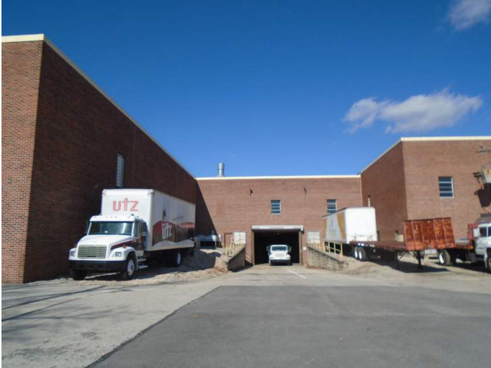
Photograph 19: The 1958 addition, showing the ell to the left, a central truck entrance, and truck-loading docks. Looking north.
