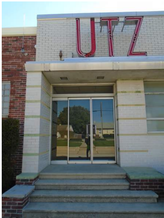
Photograph 10: Detail view of the entrance at the white brick façade, showing the original door system and masonry detailing. Looking south.
