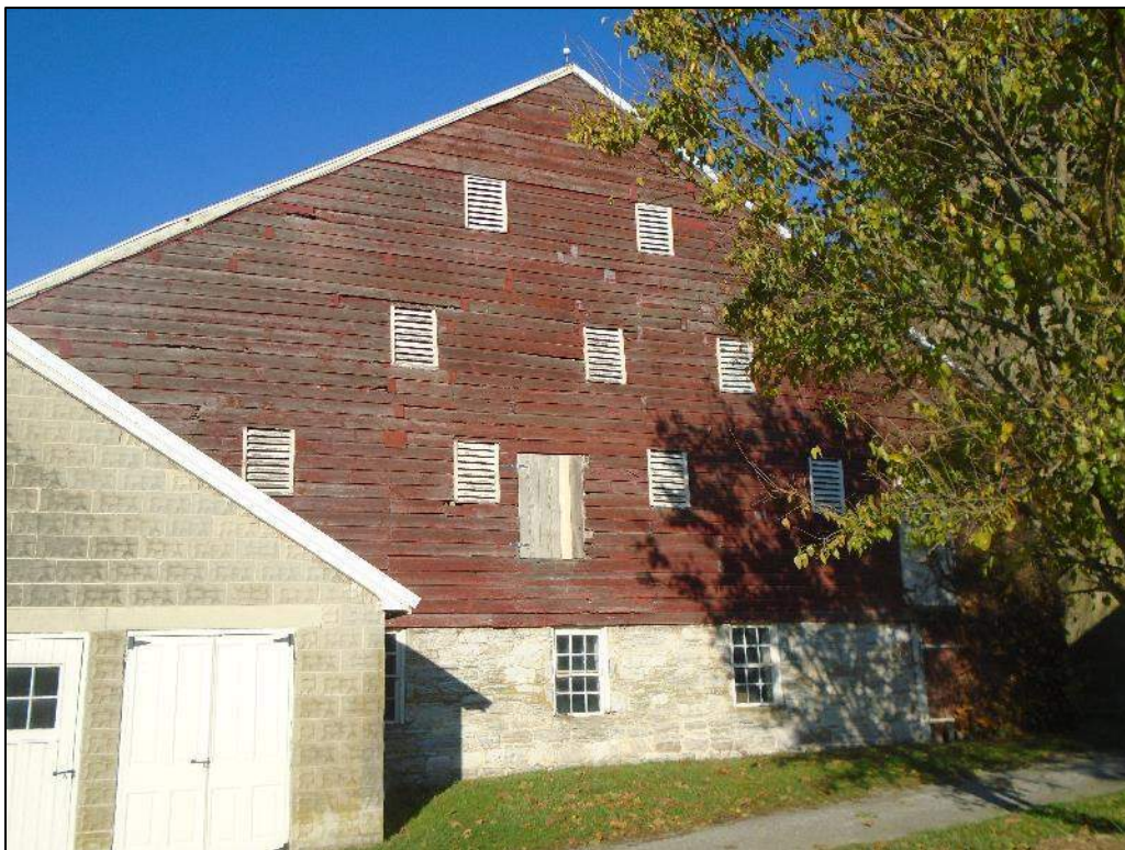
Photograph 25 – Side (east elevation) of the barn; looking west.
