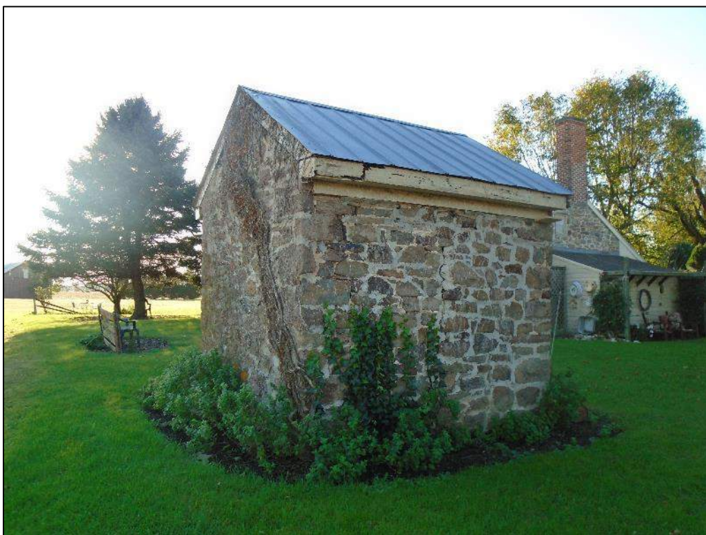
Photograph 10 – Rear (north elevation) and side (west elevation) of the smokehouse; looking southeast.
