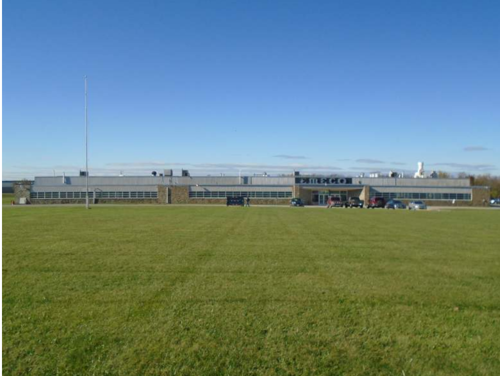
Photograph 1: Overview of the Emeco building facade (southwest), showing the original 1950s building and 1968 addition (right to left). Looking northwest.
