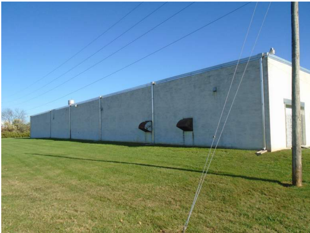
Photograph 12: The post-1971 addition, showing the northwest elevation. Looking northeast.
