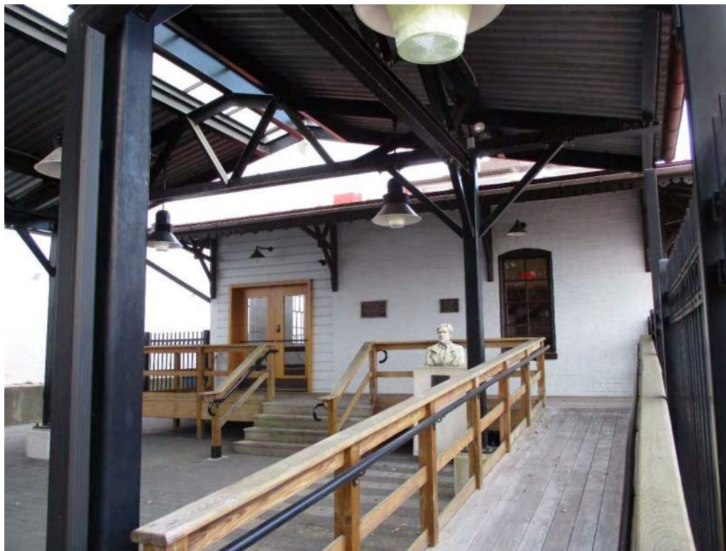
Photograph 39: View of Gettysburg Passenger Station, looking west.
