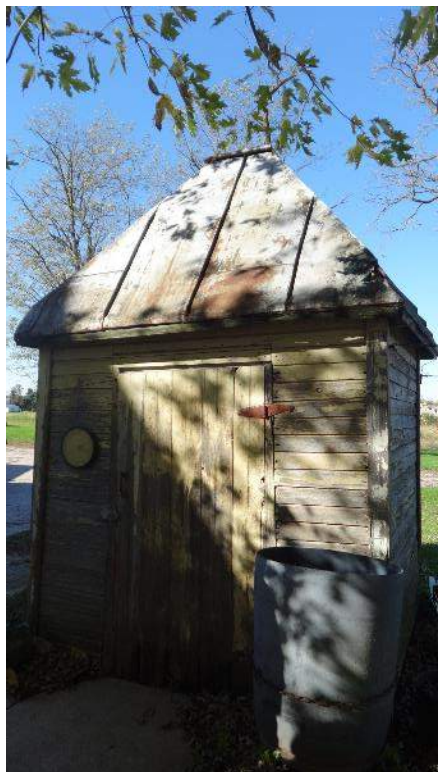
Photograph 5 – Façade (southeast elevation) of the Poist Farm pump house; looking northwest.
