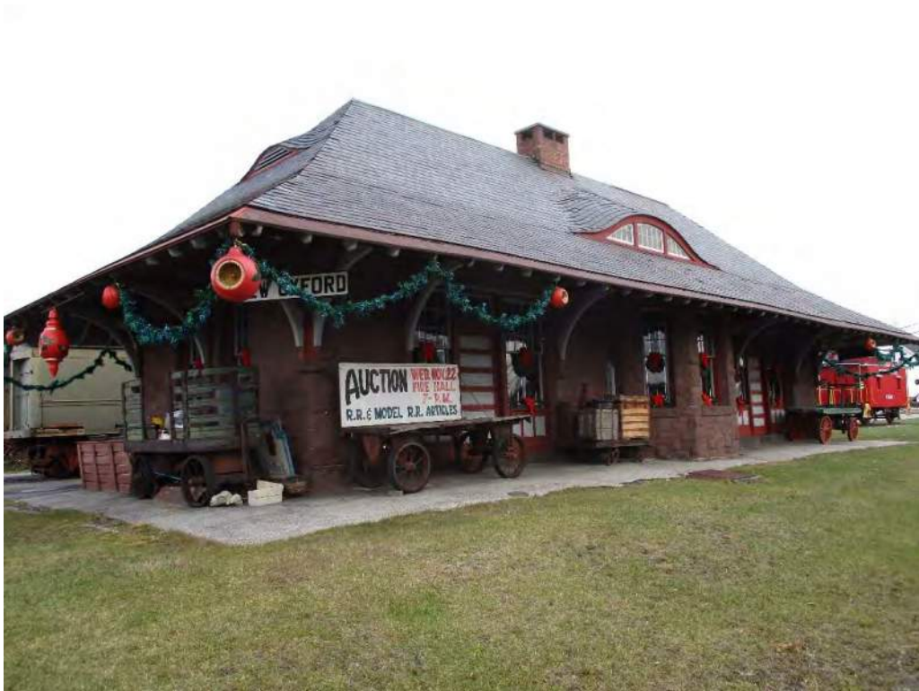
Photograph 32: View of the New Oxford Passenger Station, looking north.
