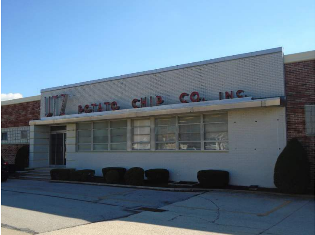
Photograph 9: The highly stylized, white brick façade at the original c. 1949 factory building. Looking southeast.
