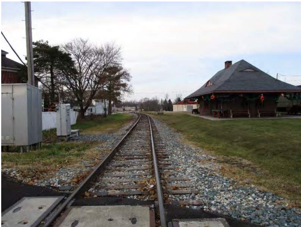
Photograph 16: View of the former Gettysburg Railroad alignment, New Oxford, from the Lincoln Way West crossing, looking northwest toward the New Oxford Passenger Station.
