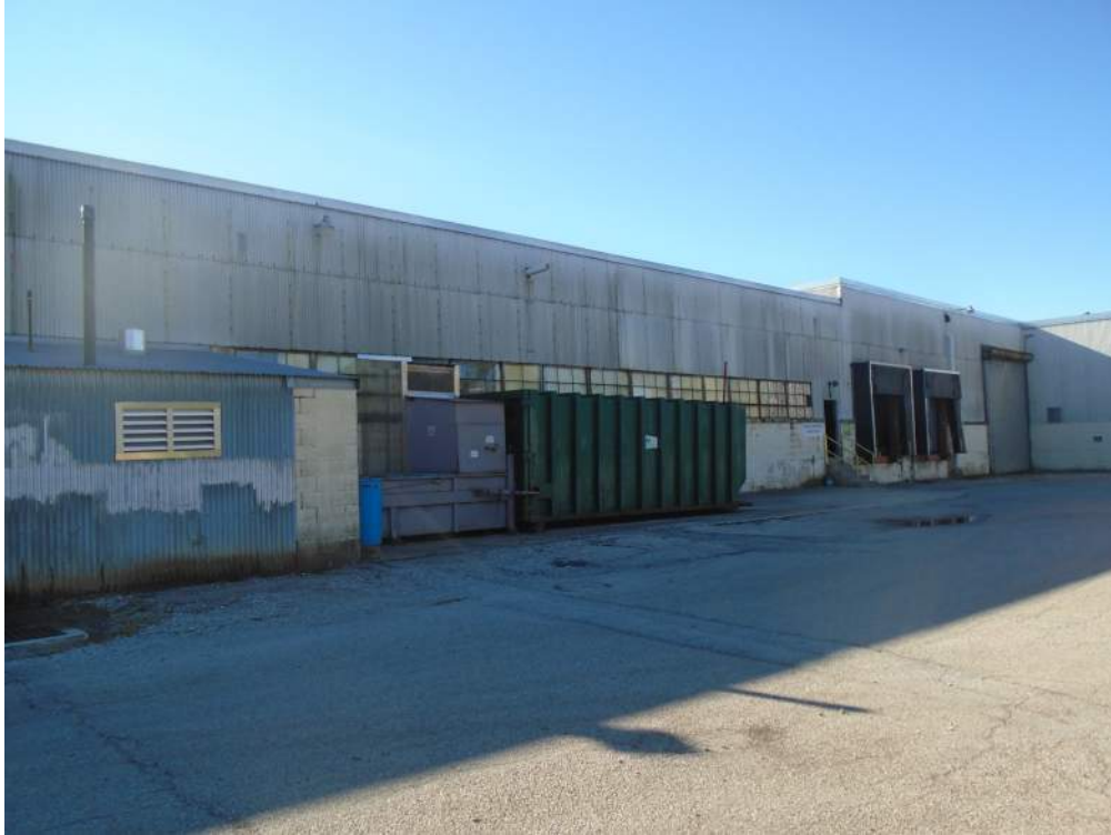
Photograph 7: Detail view of the northeast elevation of the 1950s factory building. Looking northwest.
