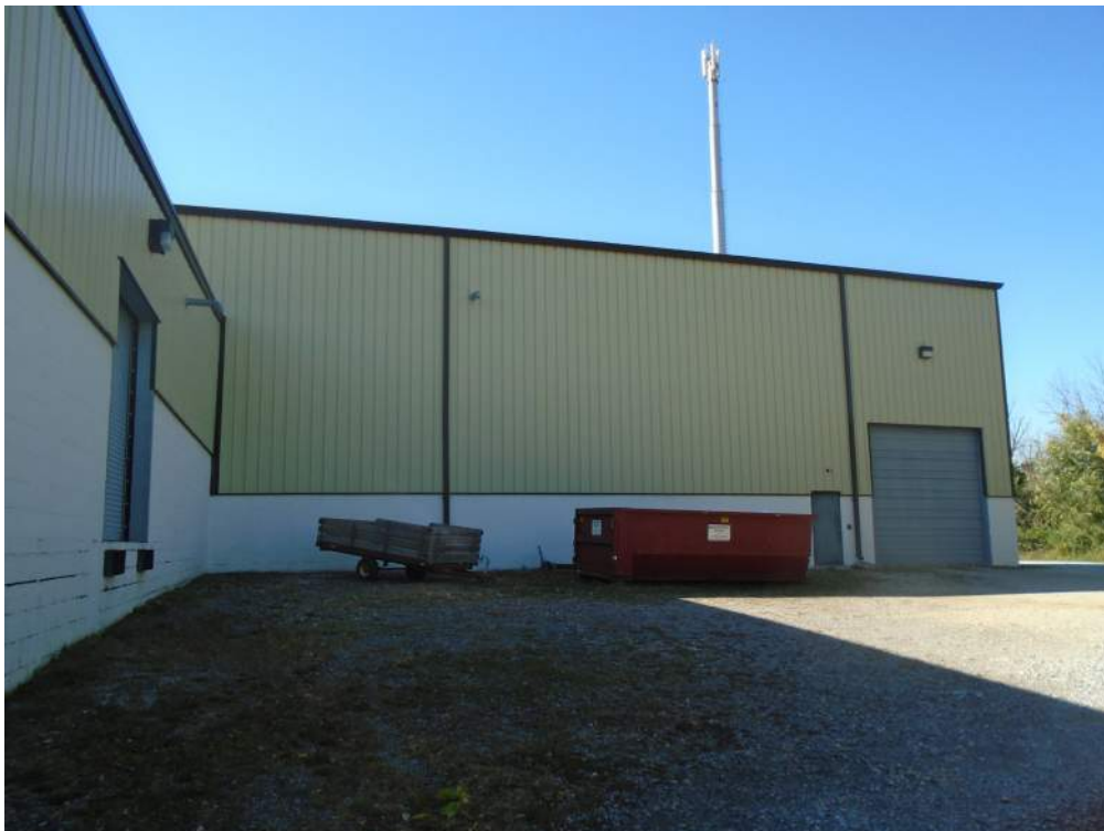
Photograph 16: The post-1971, storage addition, showing the east elevation of the western-most section. Looking west.
