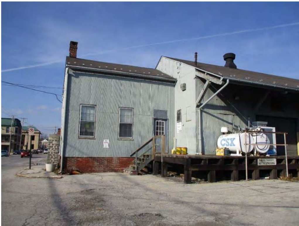
Photograph 30: View of the Western Maryland Freight Depot (Key No. 073592), looking north.
