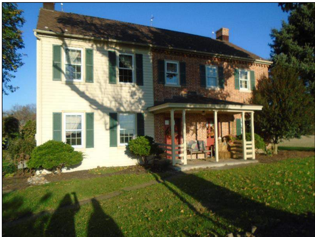
Photograph 1 – Façade (east elevation) of the dwelling; looking northwest.
