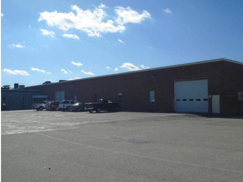
Photograph 31: The east elevation of the 1968 addition. Looking southwest.
