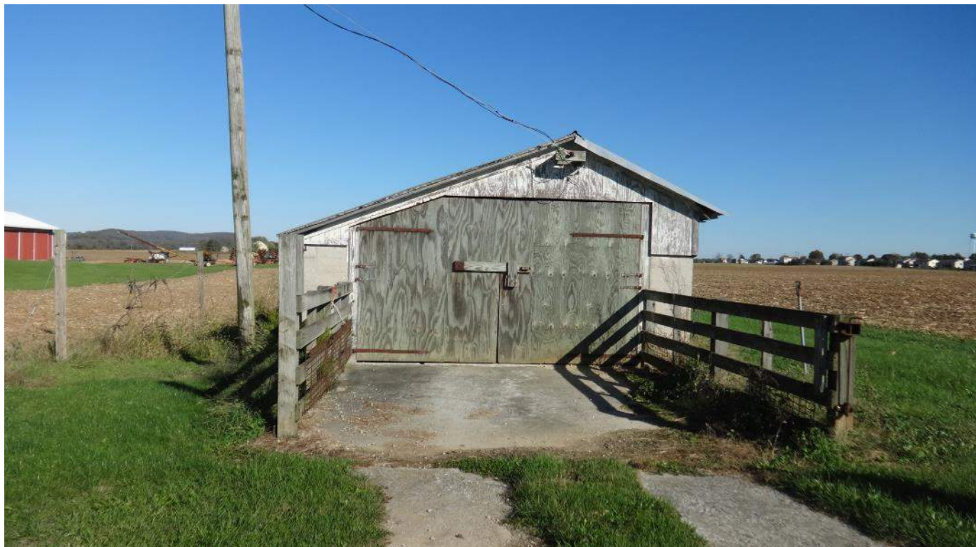
Photograph 27 – Façade (west elevation) of the Divine Chapel hog house, looking east.
