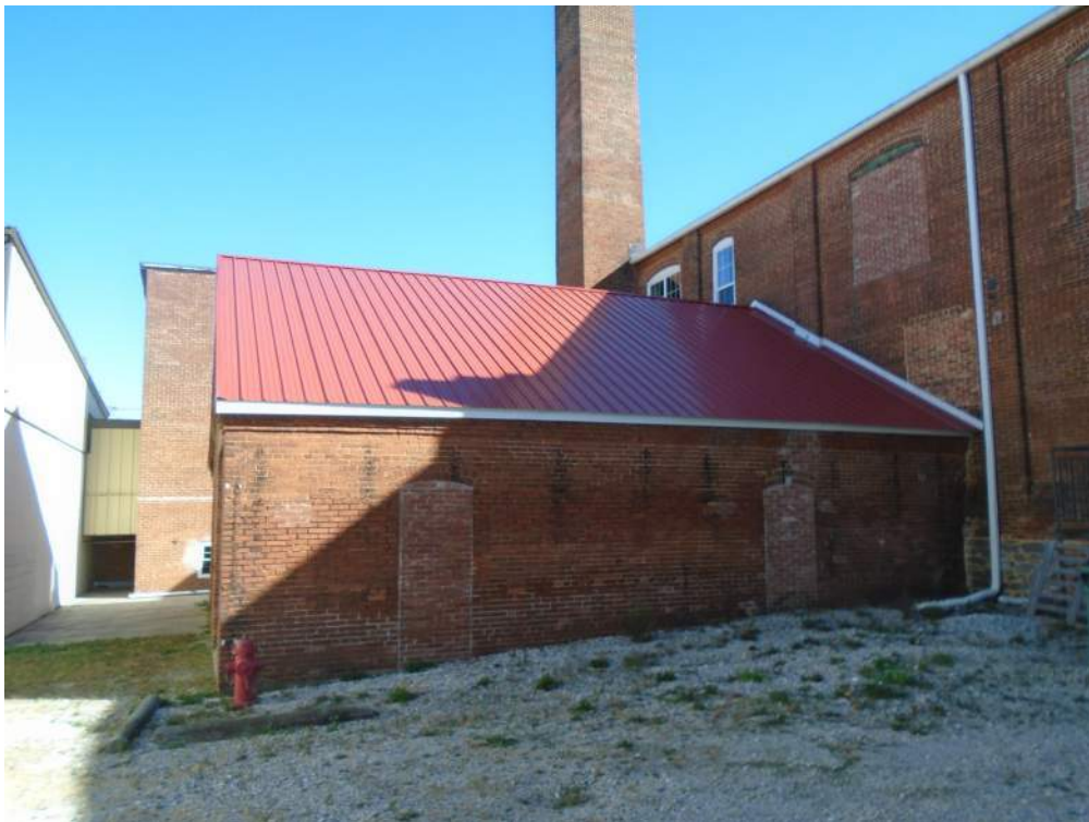
Photograph 8: The engine room ell, showing the west elevation. Looking east.
