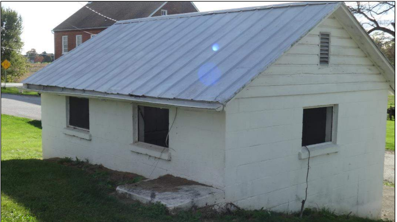
Photograph 36 – Rear (east elevation) and side (north elevation) of the Enders Farm milk house; looking southwest.
