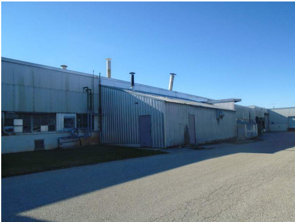
Photograph 6: The northeast elevation of the 1950s factory building, showing the two aluminum-clad, attached structures. Looking northwest.
