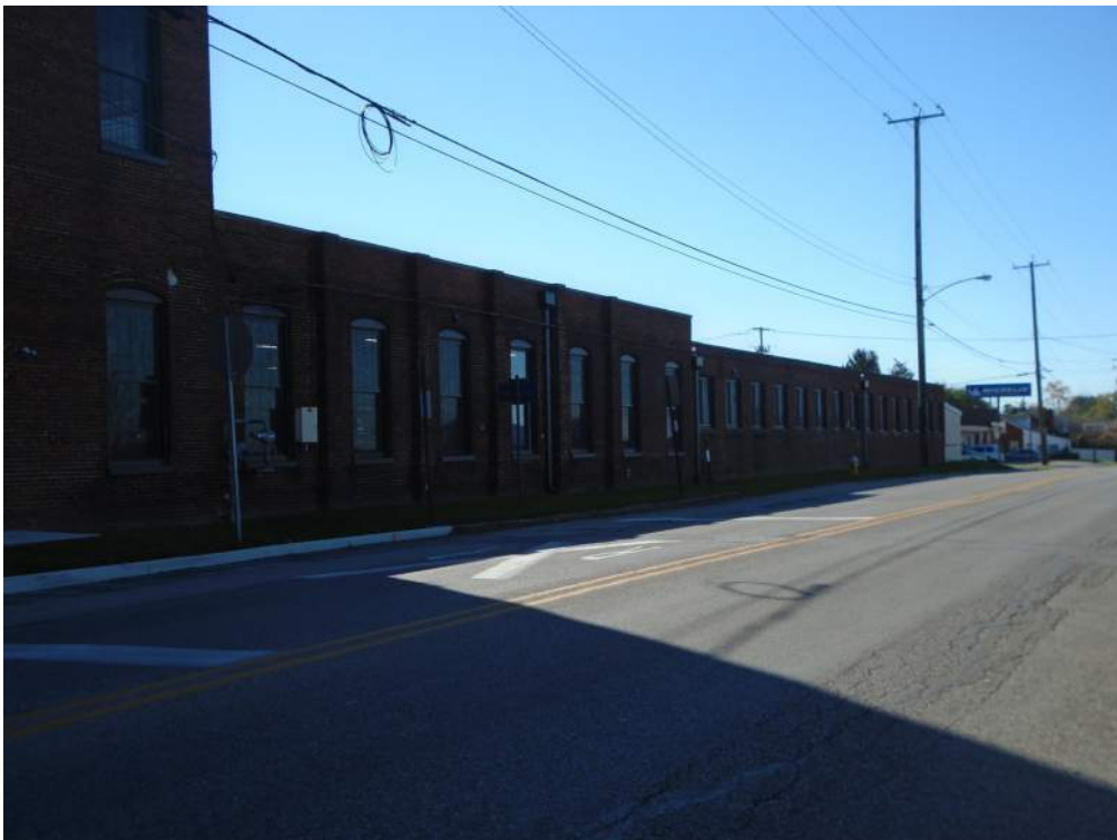
Photograph 10: North elevation of the c. 1910 and c. 1935 additions (left to right, 2017). Looking southwest.
