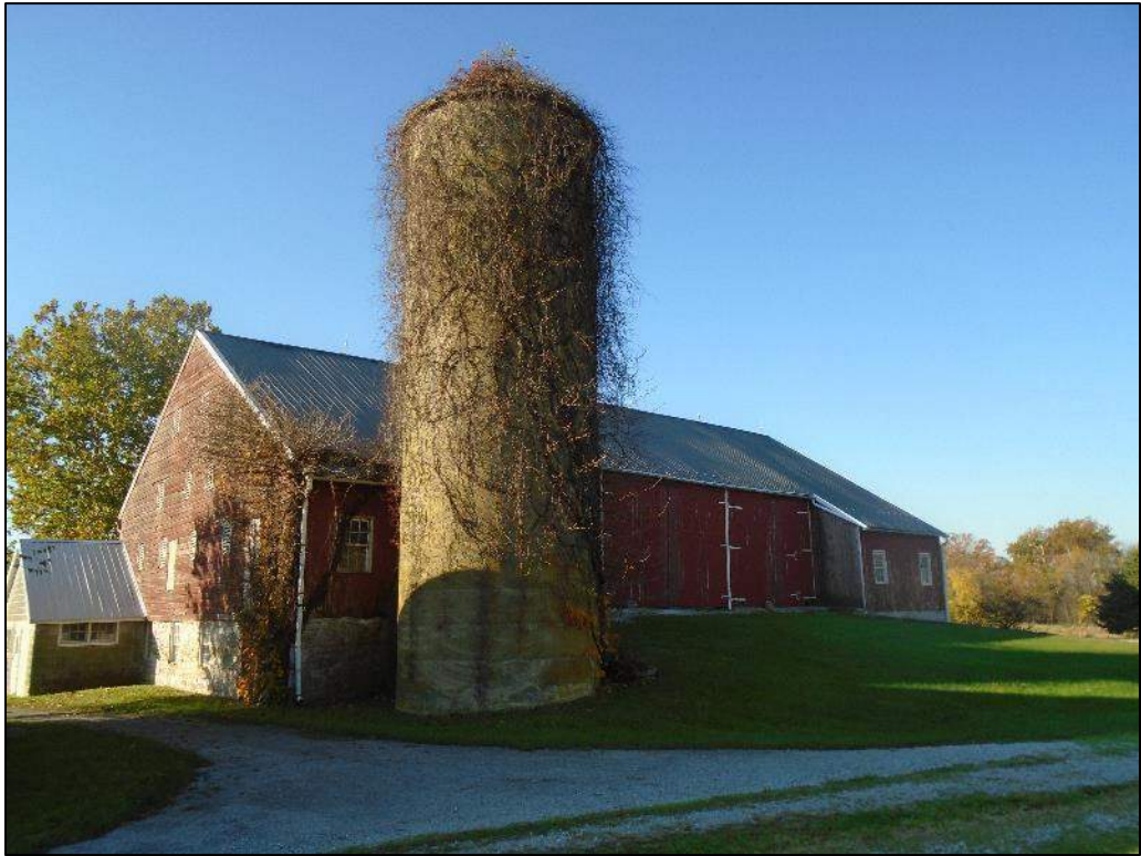
Photograph 17 – Banked (north) elevation and side (east elevation) of the barn; looking southwest.
