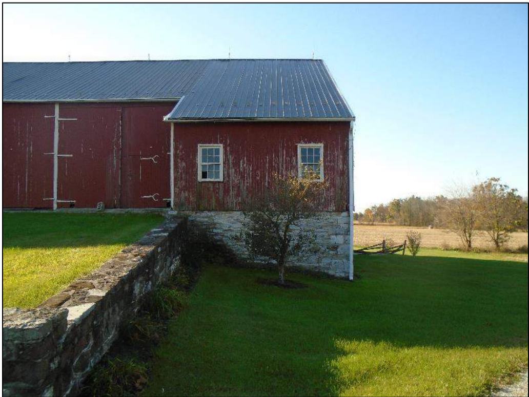
Photograph 18 – Stone retaining wall on the façade (north elevation) of the barn; looking south.
