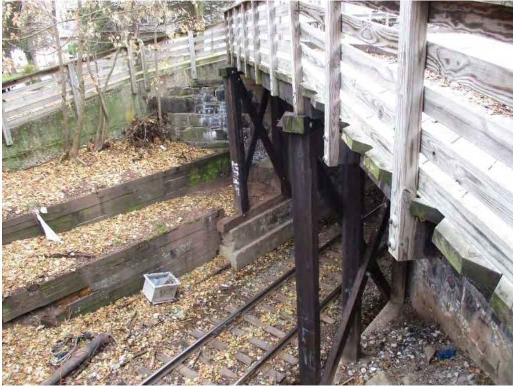
Photograph 15: View of the High Street Bridge (Key No. 083678) (Bridge 2), New Oxford, looking northwest.
