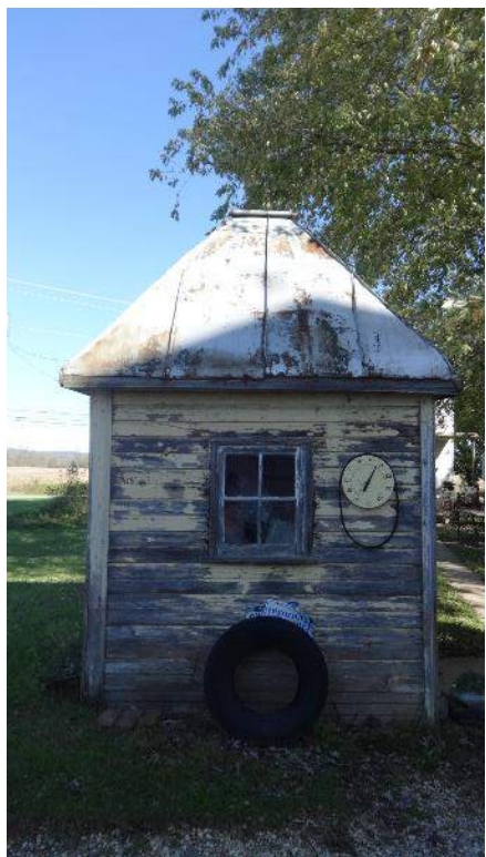
Photograph 6 – Side (southwest elevation) of the Poist Farm pump house; looking northeast.
