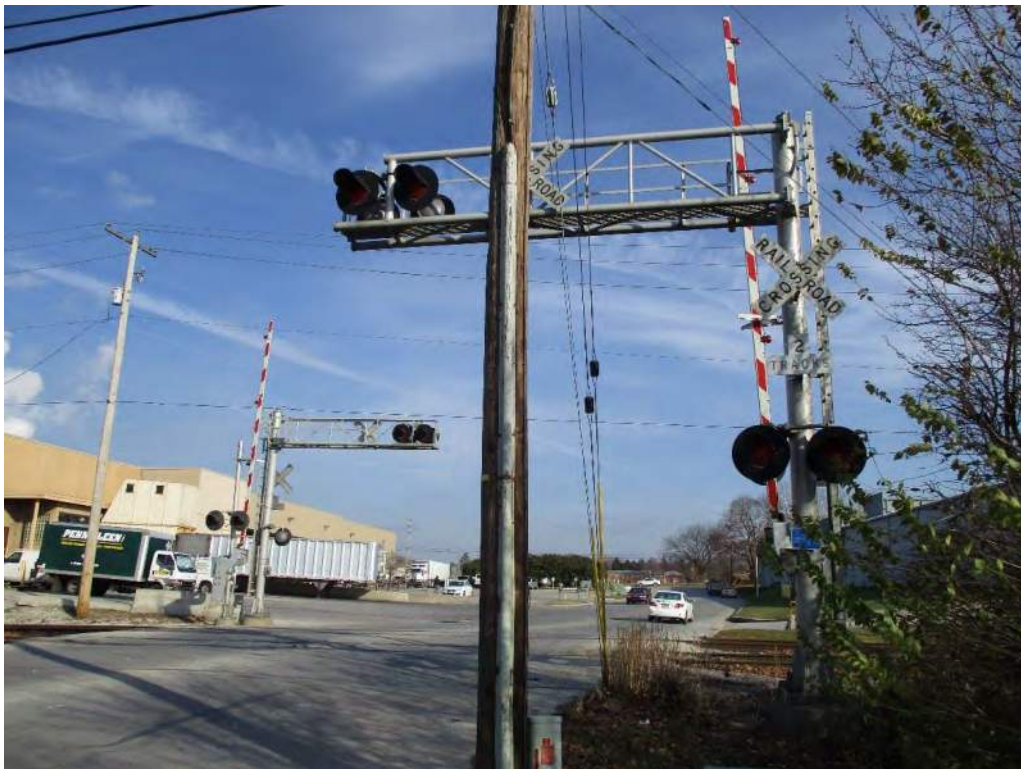
Photograph 6: View of the grade crossing signals (typical), in Hanover at the Kindig Lane crossing, looking east.
