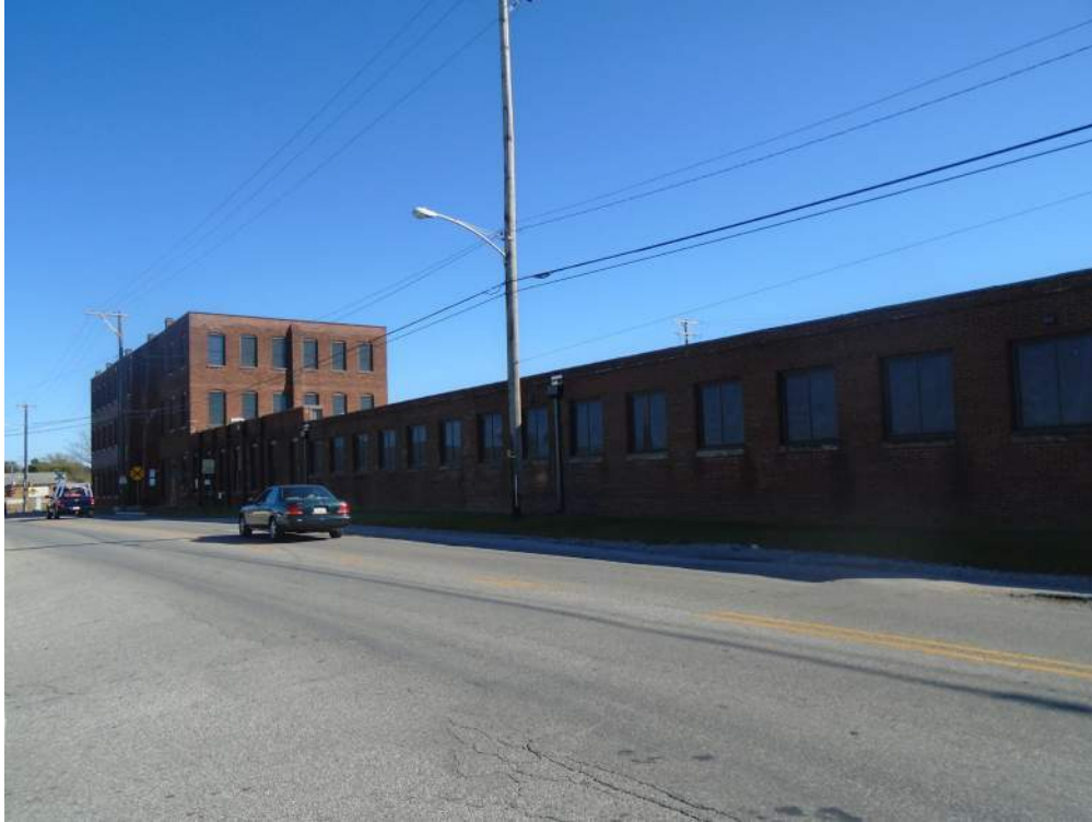
Photograph 11: North elevation of the 1892 factory, c. 1910 addition, and c. 1935 addition (left to right, 2017). Looking southeast.
