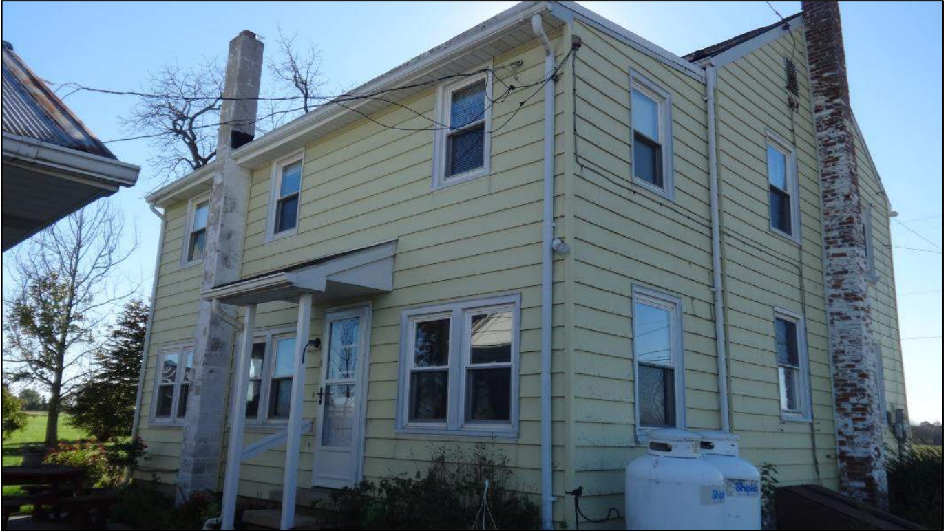
Photograph 19 – Side (north elevation) and rear (east elevation) of the Divine Chapel dwelling; looking southwest.
