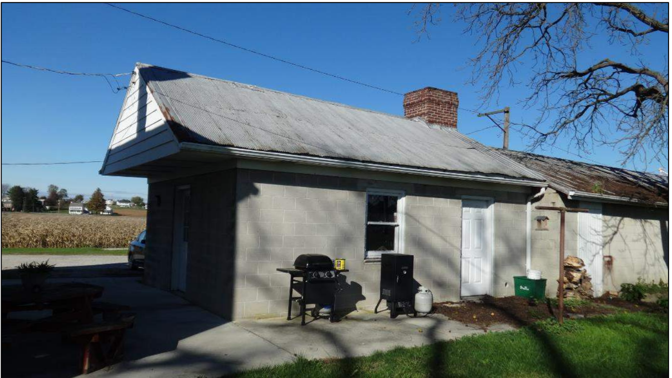
Photograph 20 – Facade (west elevation) and side (south elevation) of the Divine Chapel milkhouse; looking north.
