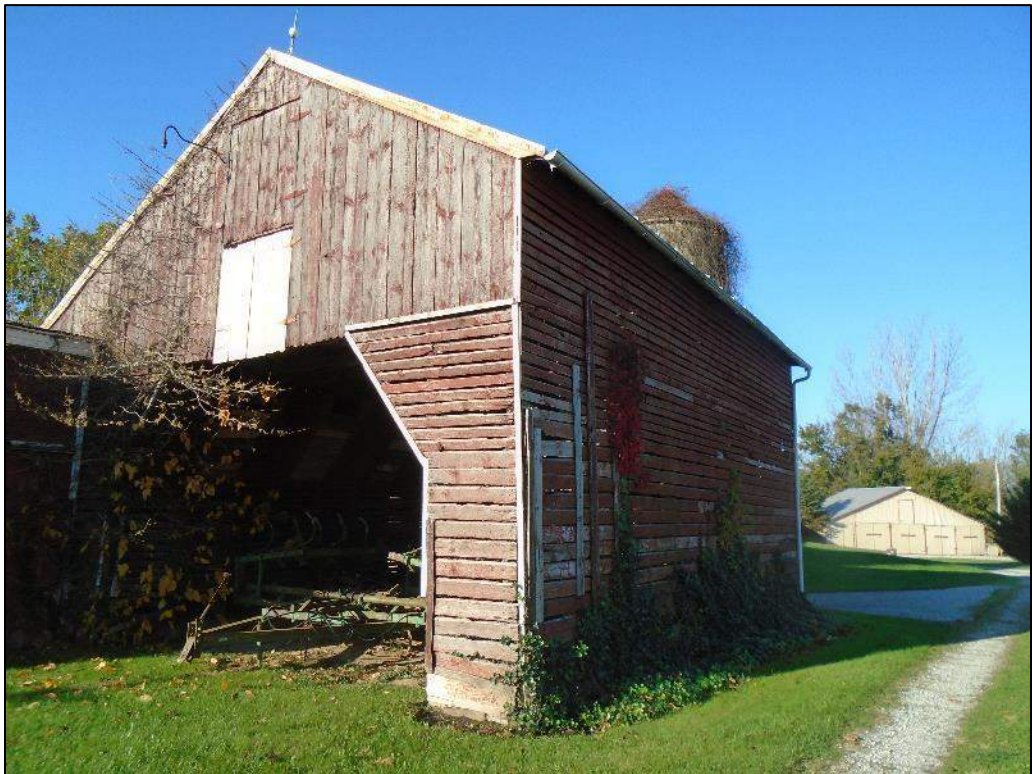
Photograph 27 – Side (north elevation) and rear (east elevation) of the drive thru corn crib; looking southwest.
