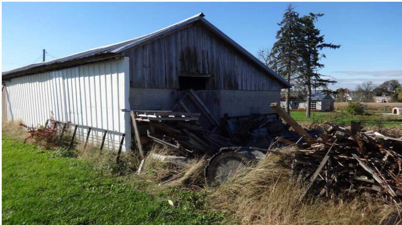
Photograph 29 – Rear (east elevation) of the Divine Chapel hog house, looking west.
