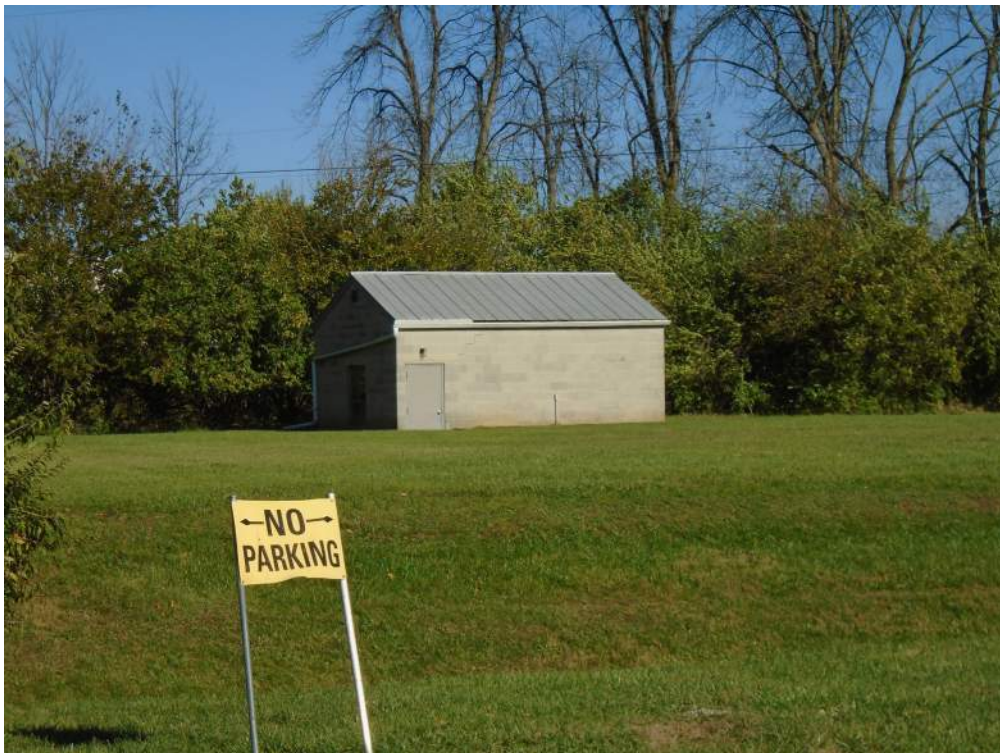
Photograph 10: The unattached, CMU building east of the factory complex. Looking east.
