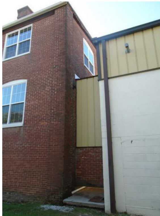
Photograph 11: The c. 1930s ell, showing the north elevation and connection to the post-1971 additions at right. Looking southwest.
