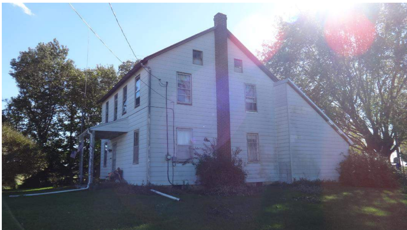
Photograph 4 – Side (northwest elevation) of the Poist Farm dwelling; looking southeast.
