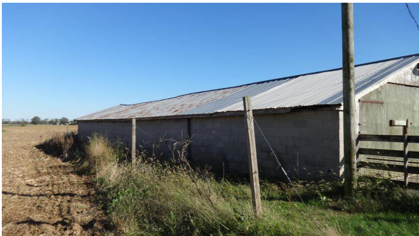
Photograph 30 – Side (south elevation) of the Divine Chapel hog house, looking northeast.
