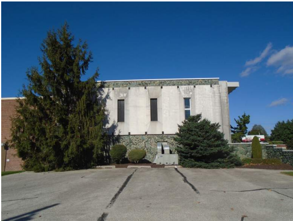
Photograph 22: The south elevation of the 1971 addition from the adjacent parking lot, showing the stone-clad retaining wall and steps at the far right. Looking north.
