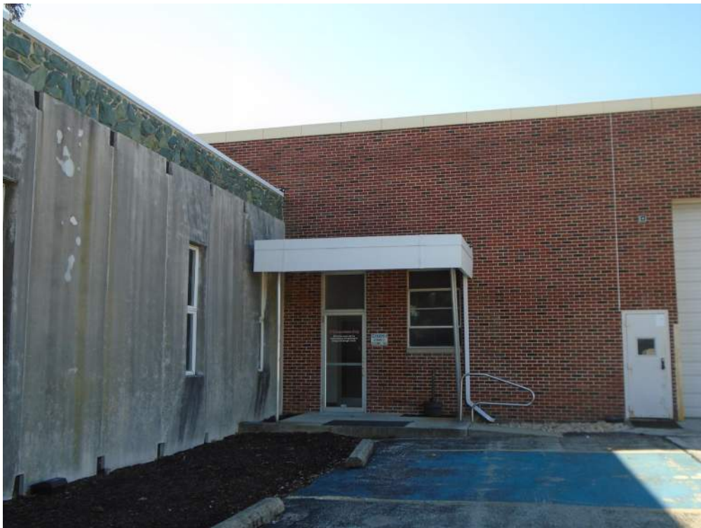
Photograph 30: View of the intersection of the 1971 addition (the north elevation at left) and 1968 addition (the east elevation at left), showing the metal canopy at the corner. Looking west.
