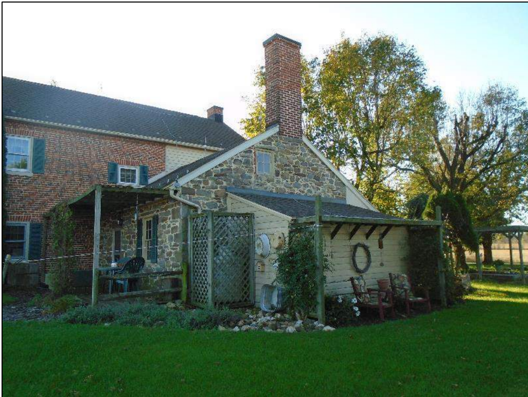
Photograph 4 – Rear elevation of the dwelling; side (north elevation) and rear (west elevation) of the summer kitchen; looking southeast.
