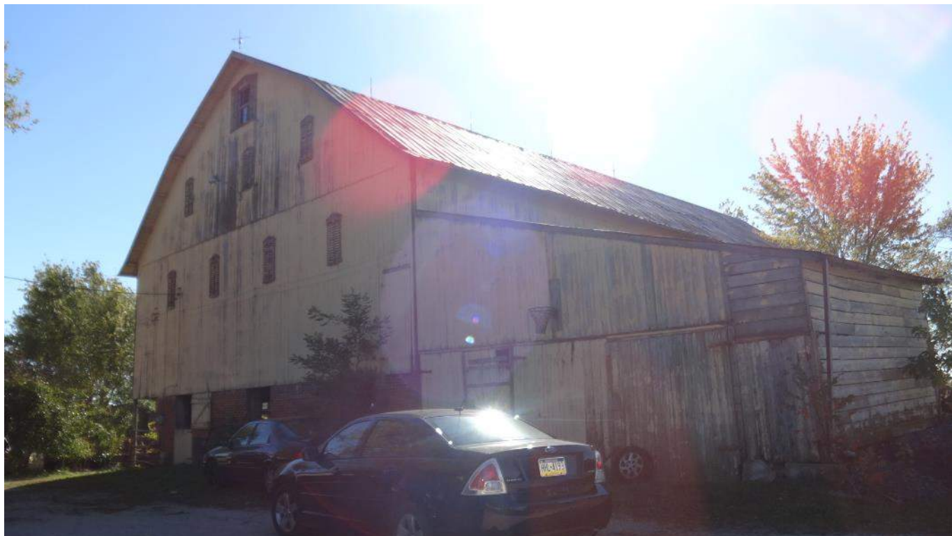
Photograph 9 – Northeast elevaton of the Poist Farm barn and addition; looking southwest.
