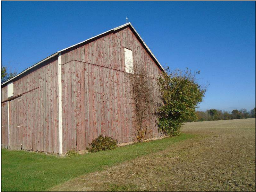
Photograph 31 – Front (south elevation) and side (east elevation) of the hay drying shed; looking northwest.
