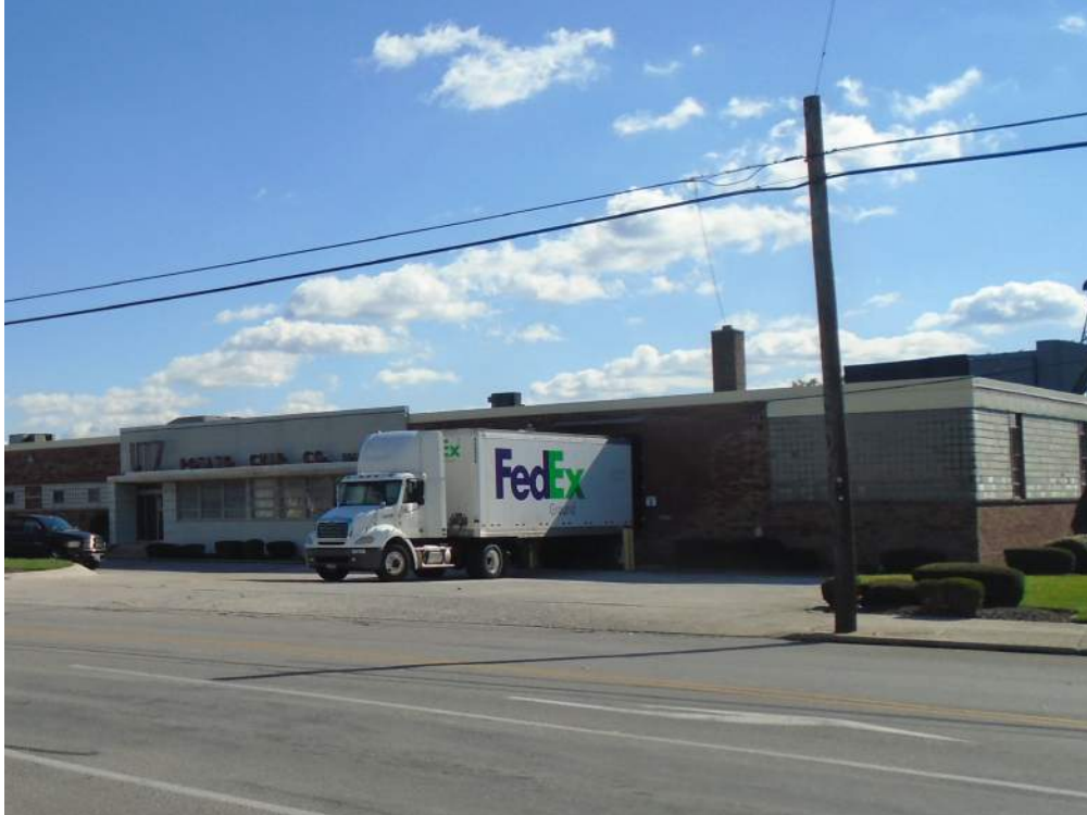
Photograph 11: View of the northwest corner of the Utz Potato Chip Co. factory building, showing the truck-loading door and glass block glazing.
