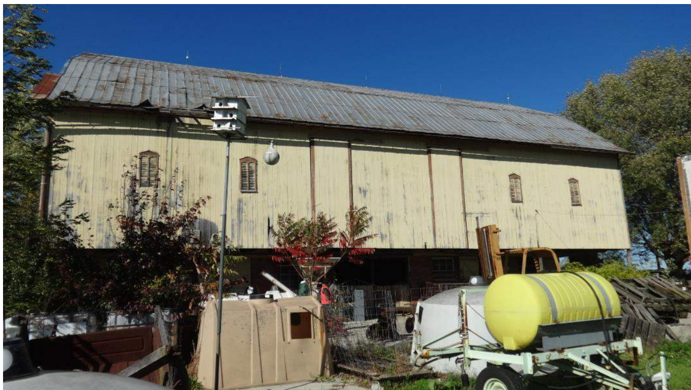
Photograph 12 – Southeast elevation of the Poist Farm barn; looking northwest.
