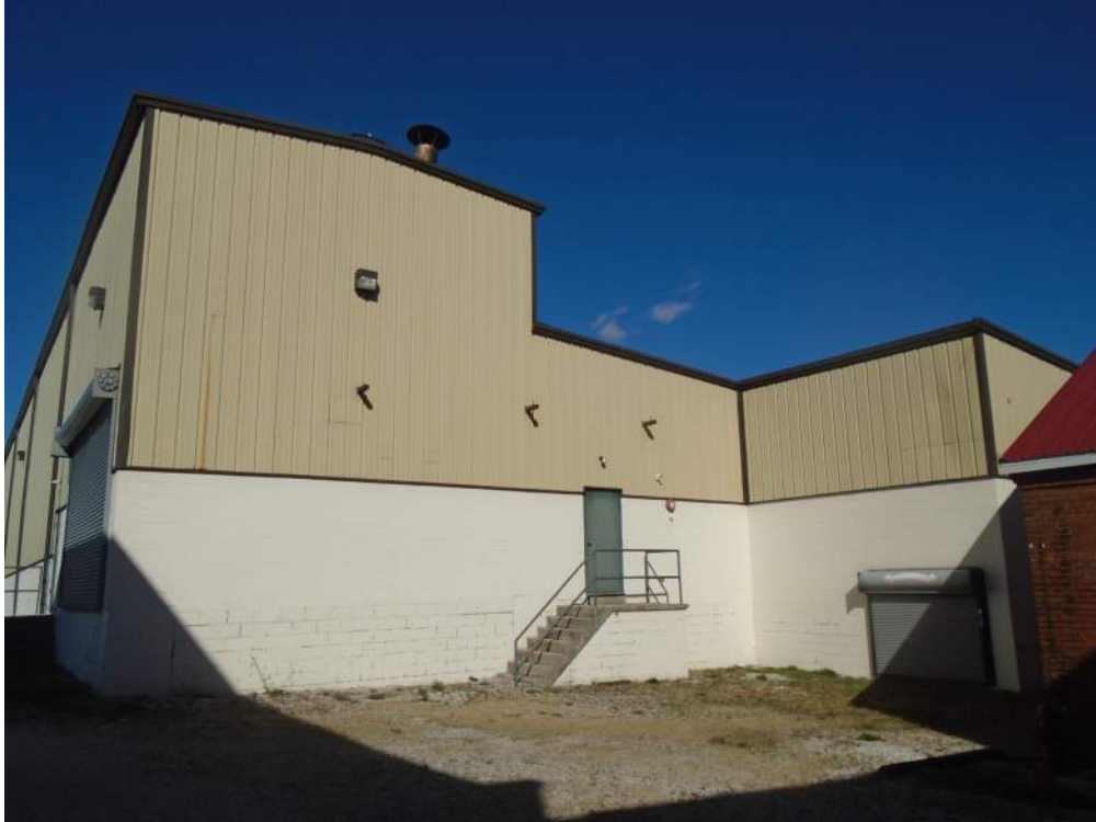
Photograph 19: The post-1971, storage addition, showing the south elevation of the west section, central wing and east or southernmost section. Looking northeast.
