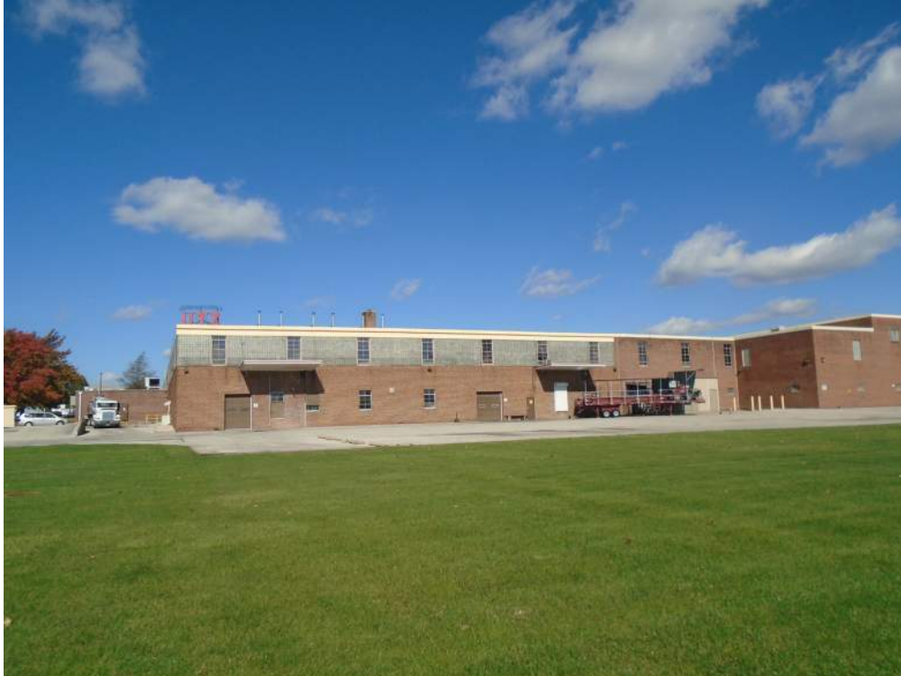
Photograph 17: The 1953 and 1956 additions (from left to right), differentiated by the termination of the glass block. The 1956 addition includes the ell with the lower roofline at the far right. Looking north.
