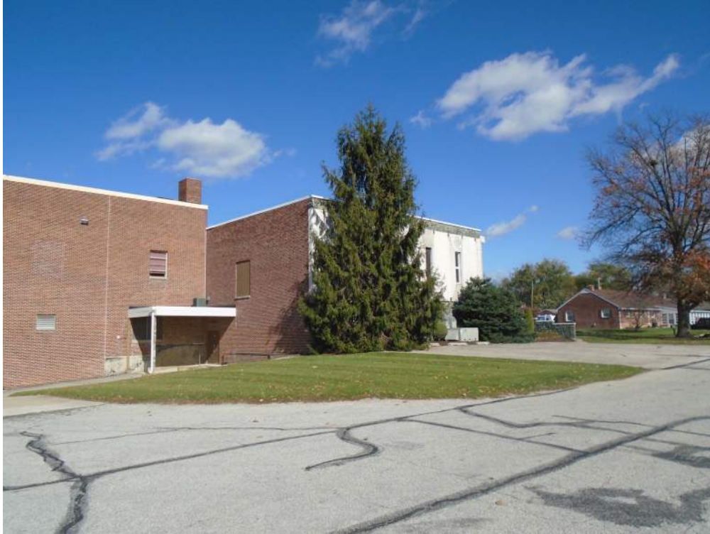
Photograph 21: The 1967 and 1971 additions (from left to right). Looking northeast.
