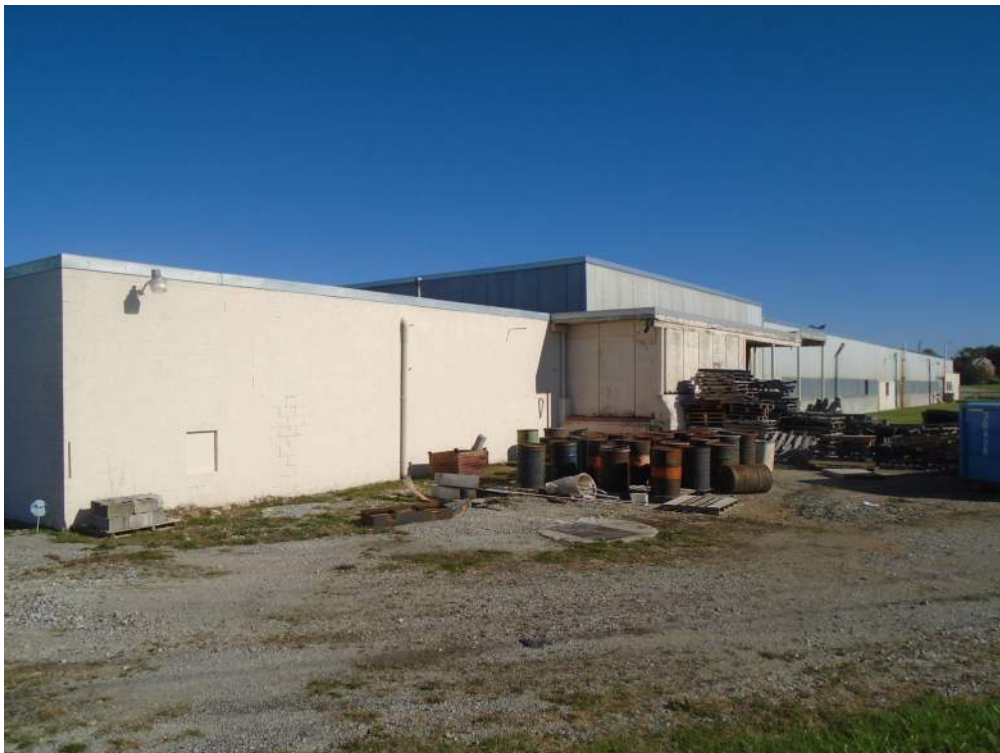
Photograph 16: The 1968 addition, showing the southwest elevation including the CMU structure at the far left. Looking southeast.
