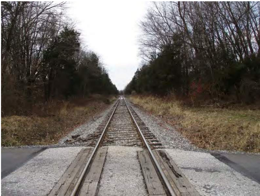
Photograph 18: View of the former Gettysburg Railroad alignment, outside of New Oxford, from the New Chester Road crossing, looking west.
