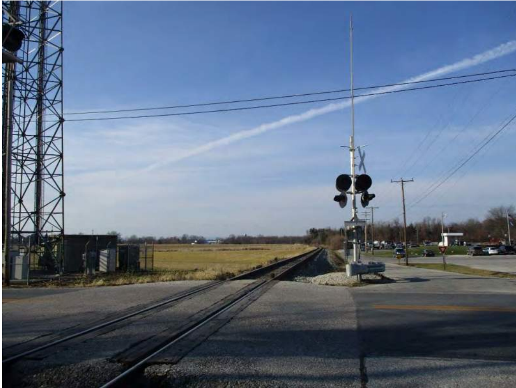
Photograph 11: View of the former Gettysburg Railroad alignment, approaching New Oxford, at the Brickyard Road crossing, looking northwest.
