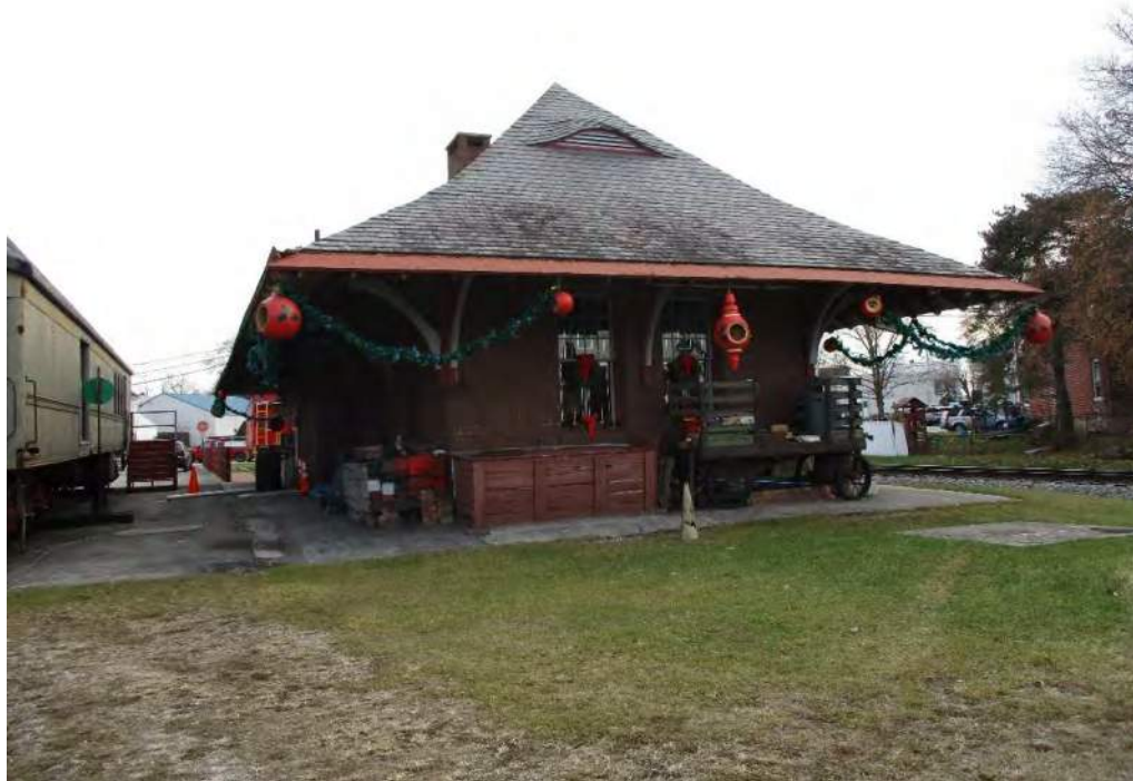
Photograph 35: View of the New Oxford Passenger Station, looking southeast.
