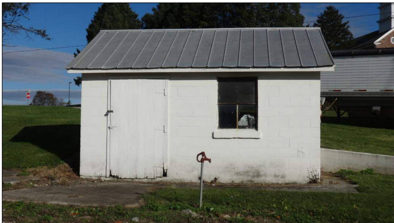
Photograph 34 – Façade (west elevation) of the Enders Farm milk house; looking east.
