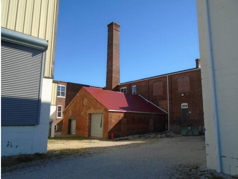
Photograph 7: The engine room ell, showing the north and west elevations. Looking southeast.
