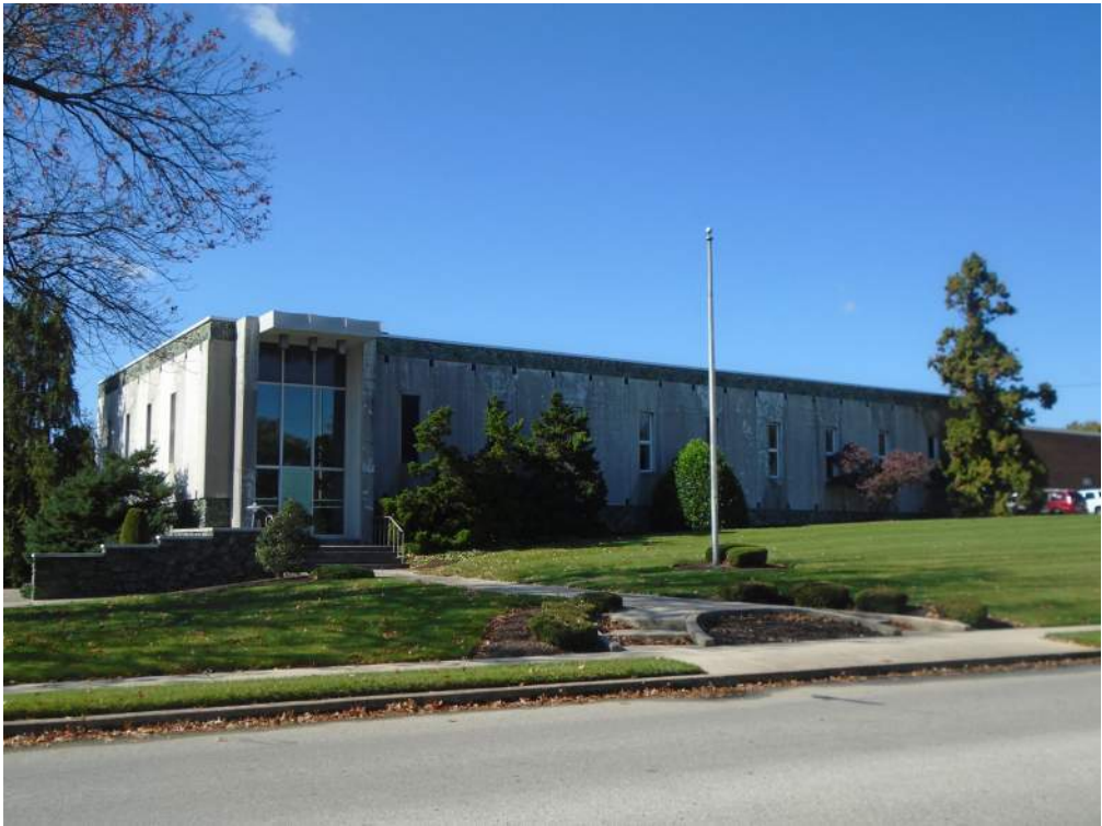
Photograph 24: The 1971 corporate office addition, showing the retaining wall at the left, half-circle path from the sidewalk, and east elevation. Looking west.
