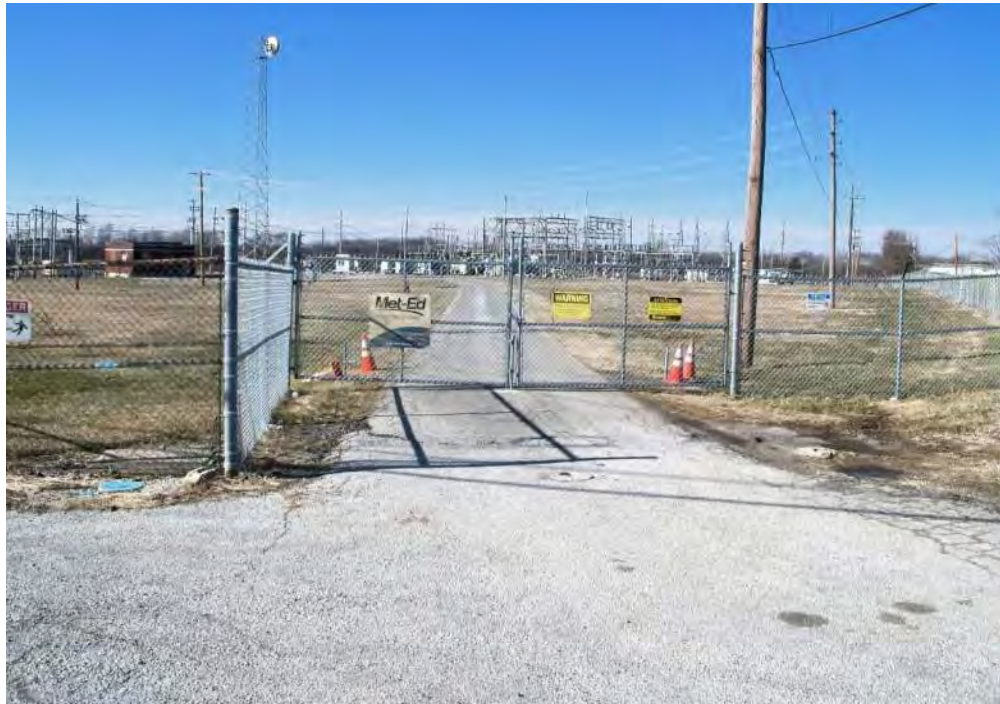
35. VIEW OF MET-ED SUBSTATION LOOKING NORTHWEST
