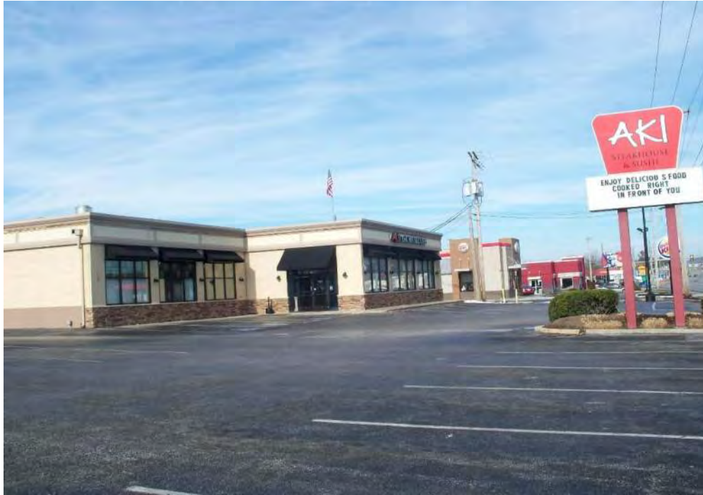
53. VIEW OF AKI BUILDING (FORMERLY LIBERTY NISSAN) LOOKING NORTHWEST
