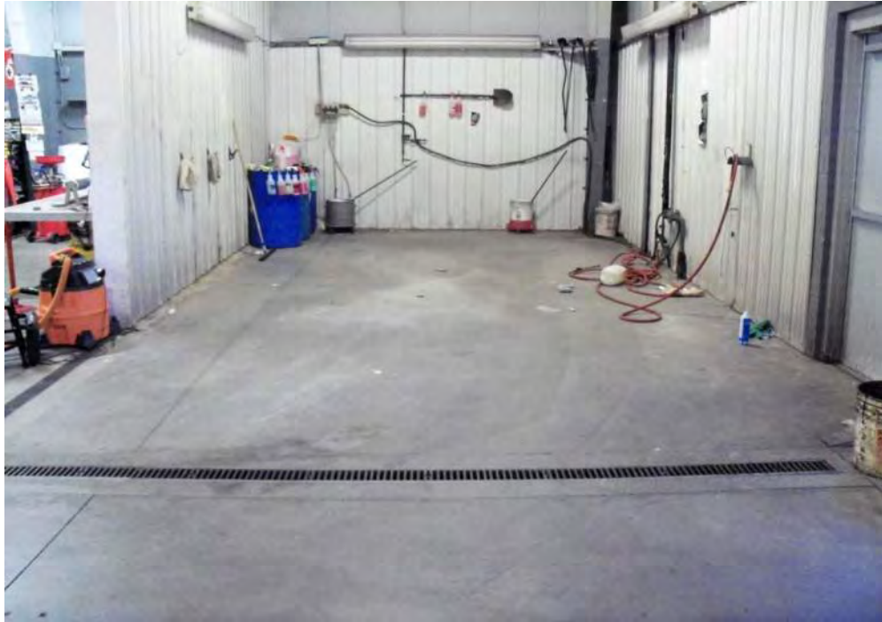
47. VIEW OF CLEANING BAY WITH DRAIN IN HANOVER NISSAN
