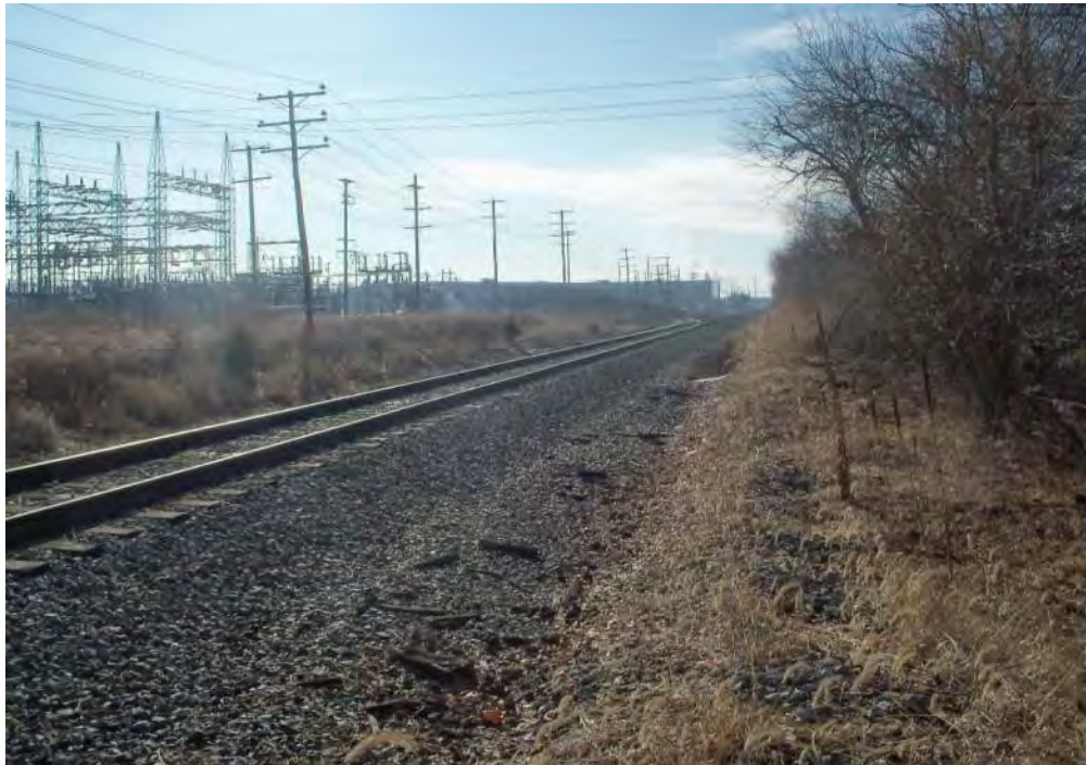
38. VIEW OF CSX RAIL LINE LOOKING SOUTH-SOUTHEAST
