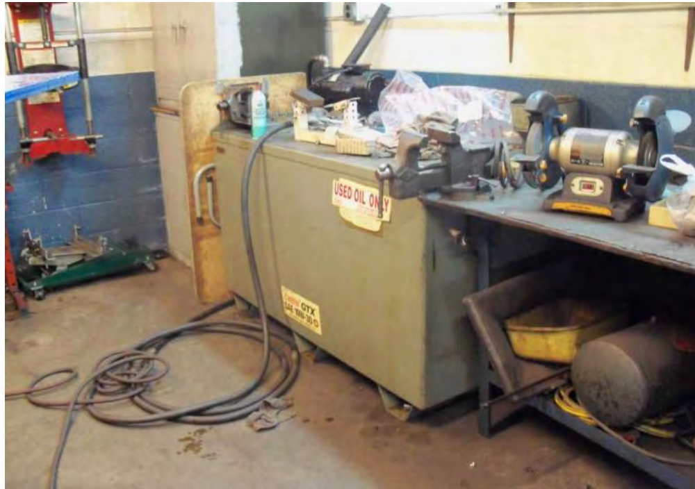
45. VIEW OF USED MOTOR OIL AST AT HANOVER NISSAN
