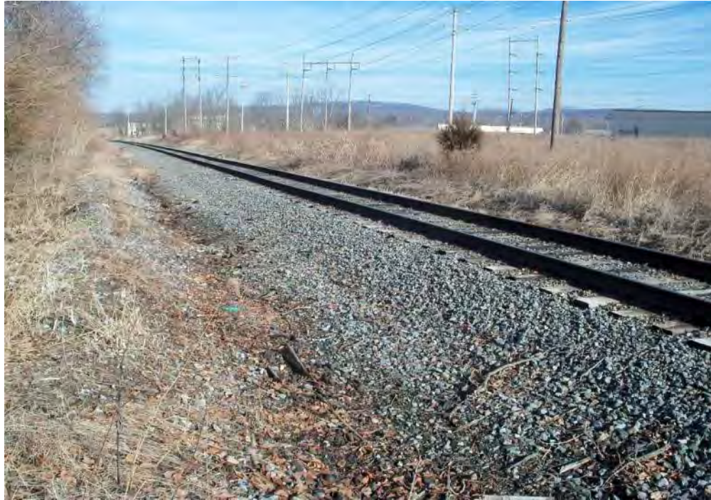
39. VIEW OF CSX RAIL LINE LOOKING NORTH FROM PROJECT AREA
