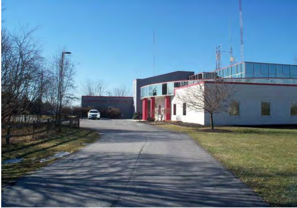
29. VIEW OF WYCR-FM BUILDING ON BARE DEVELOPMENT LP PROPERTY, LOOKING WEST
