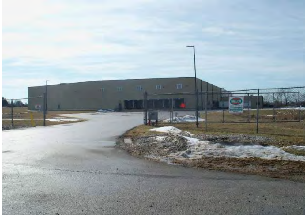
33. VIEW OF MILLER CHEMICAL BUILDING LOOKING SOUTHWEST
