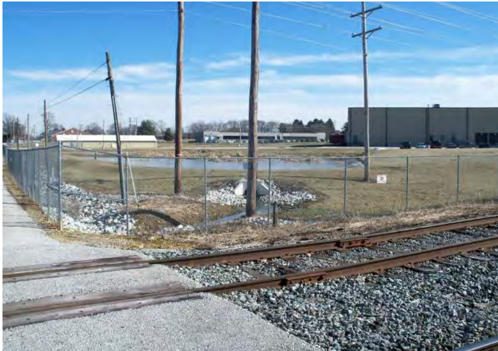
34. VIEW OF STORMWATER BASIN AND SURFACE WATER DISCHARGE ON MILLER CHEMICAL PROPERTY
