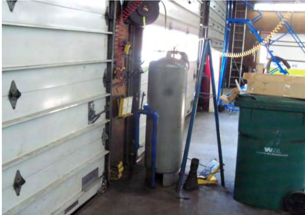
7. VIEW OF HYDRAULIC OIL TANK ASSOCIATED WITH IN-GROUND LIFT
