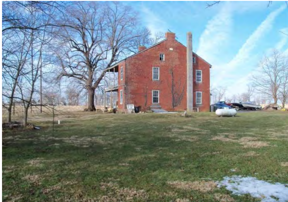
28. VIEW OF BACK OF FARM HOUSE, PROPANE TANK VISIBLE
