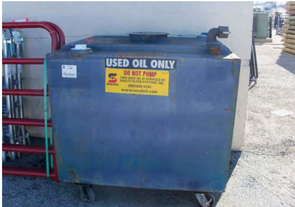
51. VIEW OF USED MOTOR OIL TANK AT TRACTOR SUPPLY
