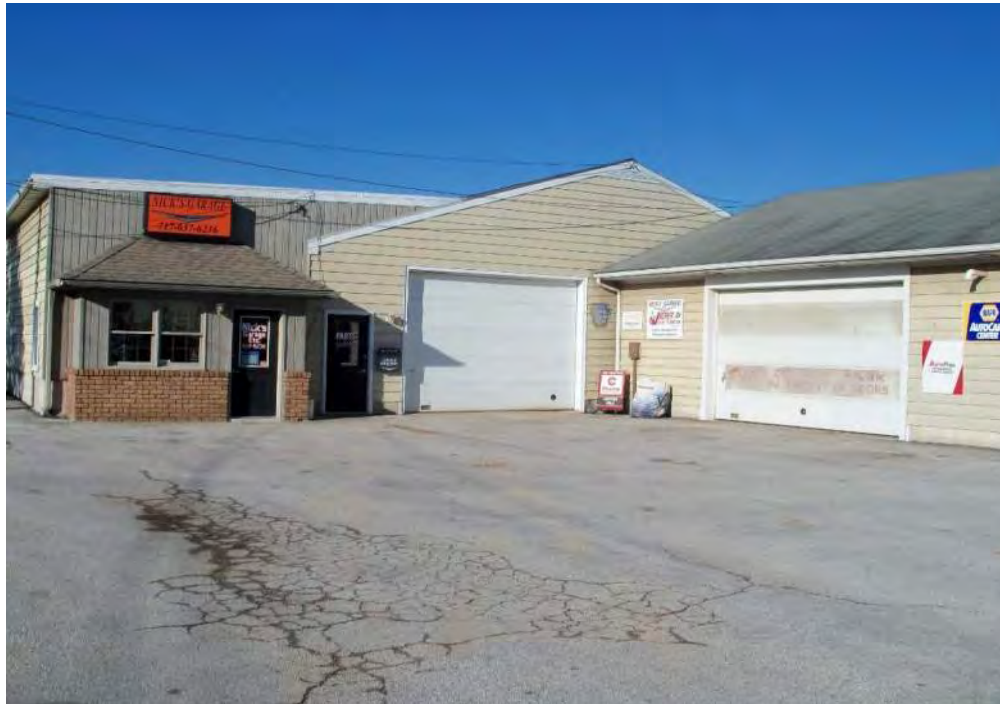
3. VIEW OF NICK'S GARAGE EXTERIOR, LOOKING NORTH
