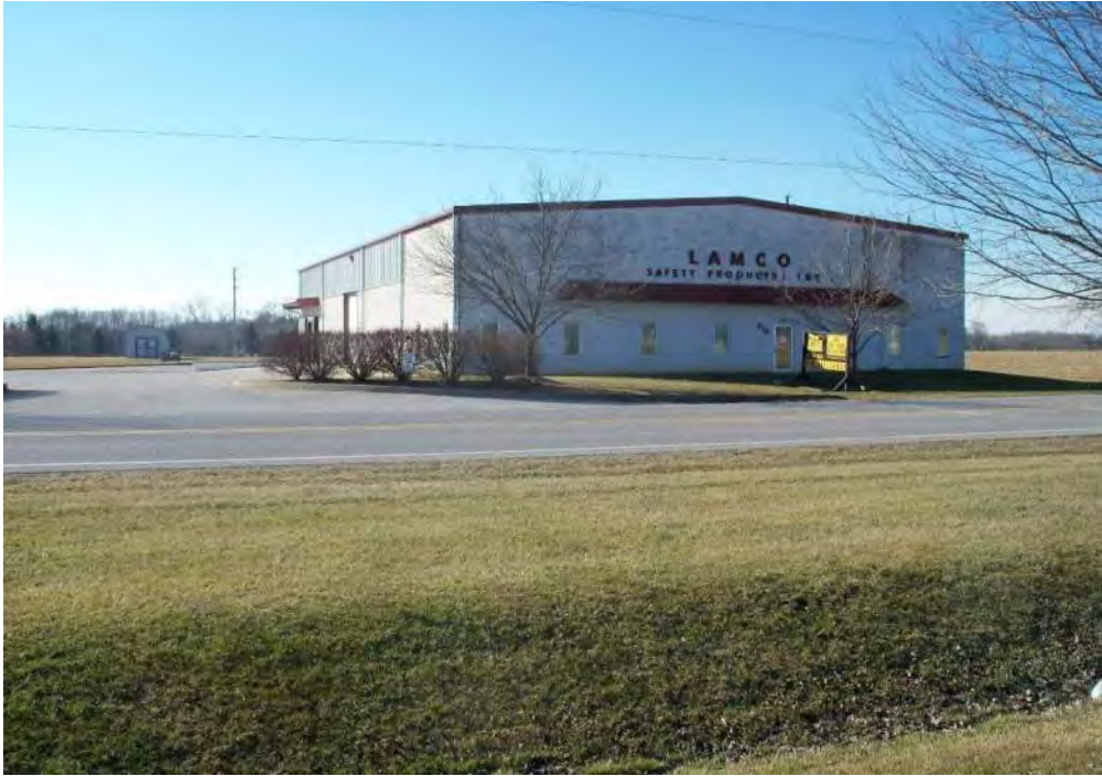
11. VIEW OF VACANT LAMCO BUILDING, LOOKING WEST
