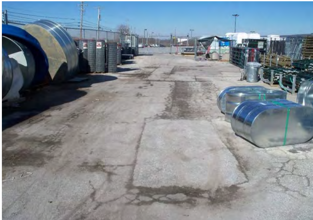
52. VIEW OF ABNORMAL CUT-OUTS IN TRACTOR SUPPLY STORAGE AREA
