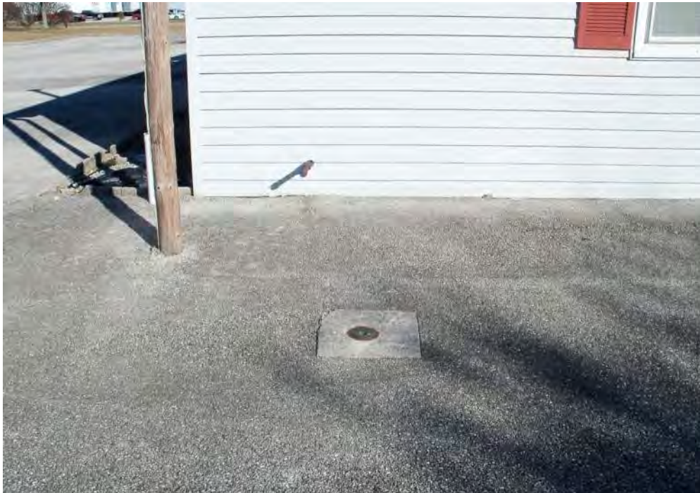
12. VIEW OF POTENTIAL FILL PORT
