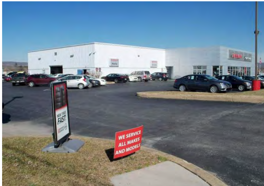
40. VIEW OF HANOVER NISSAN BUILDING LOOKING NORTHWEST
