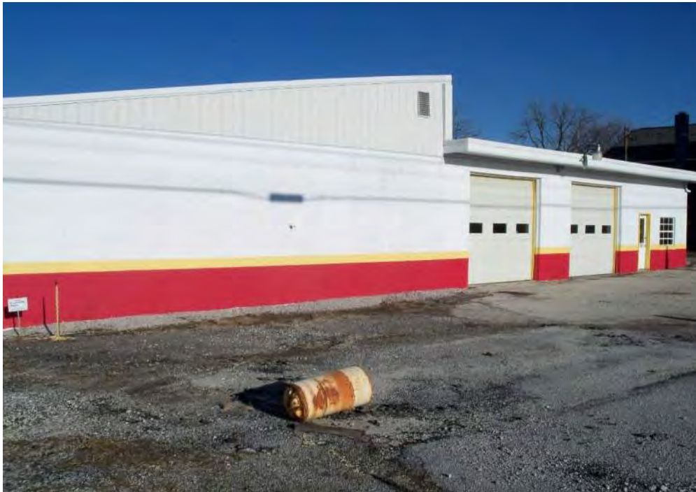
8. VIEW OF FORMER MUMMERT'S AUTO BUILDING, LOOKING NORTHEAST
