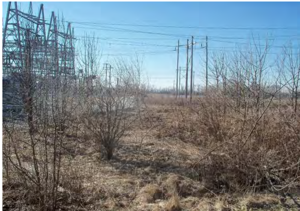
36. VIEW OF AREA BETWEEN PROPOSED PROJECT AREA AND SUBSTATION LOOKING SOUTHWEST
