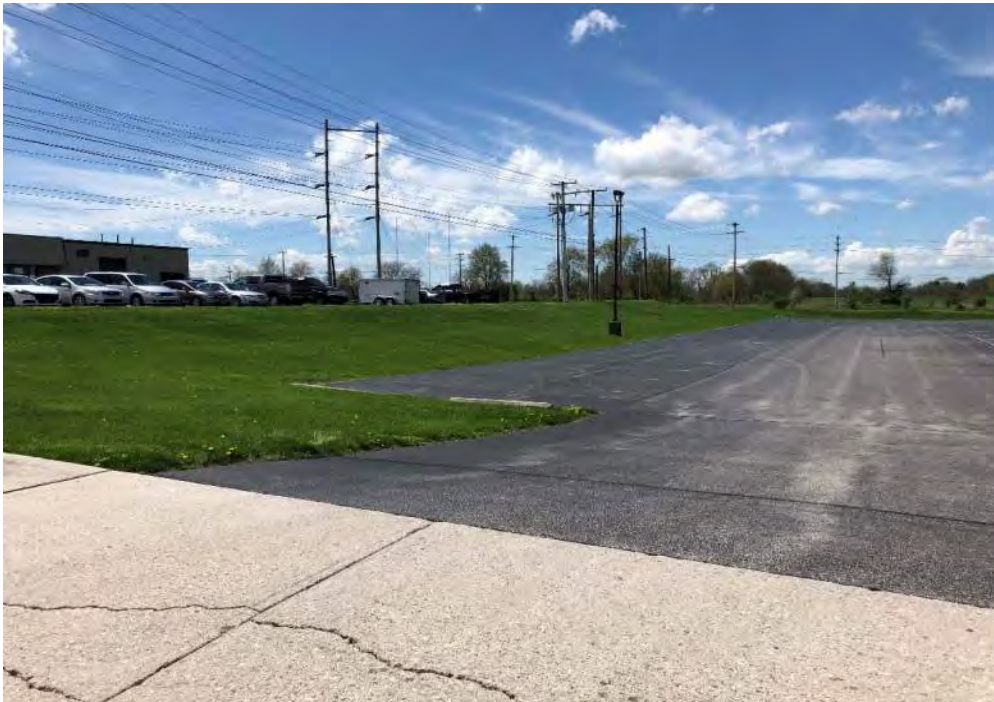
42. VIEW OF FAMILY FIRST PARKING LOT LOOKING TOWARDS PROJECT AREA
