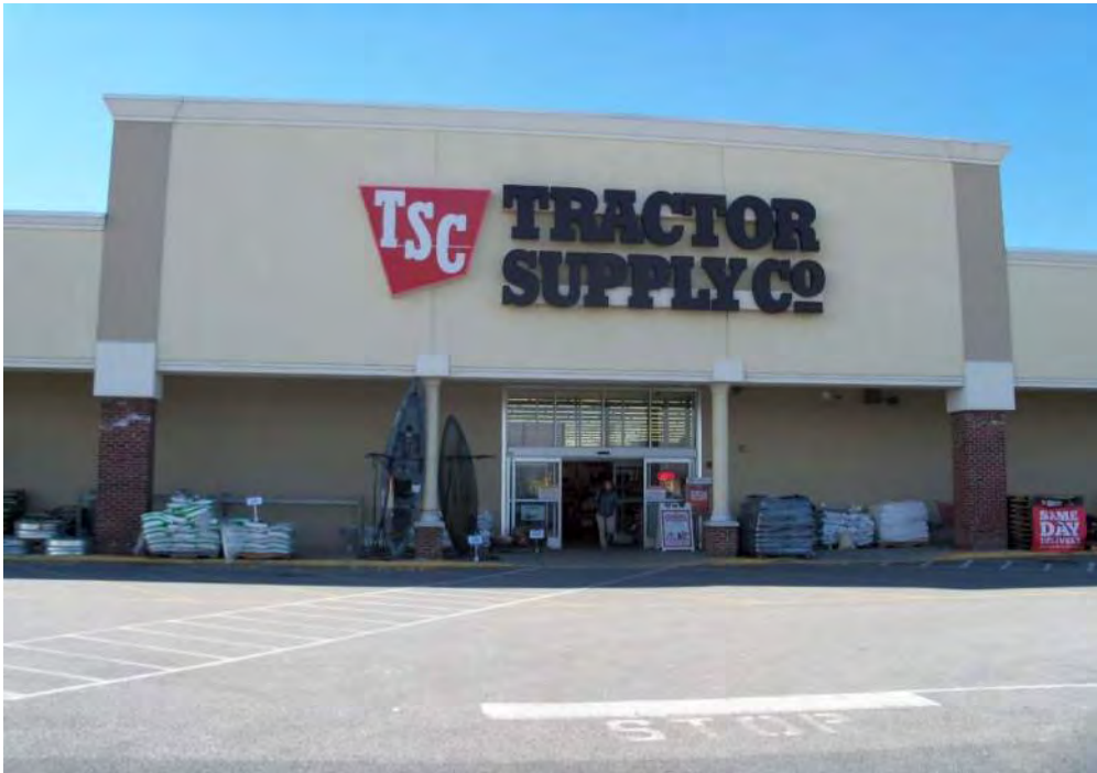
50. VIEW OF TRACTOR SUPPLY BUILDING LOOKING SOUTHWEST
