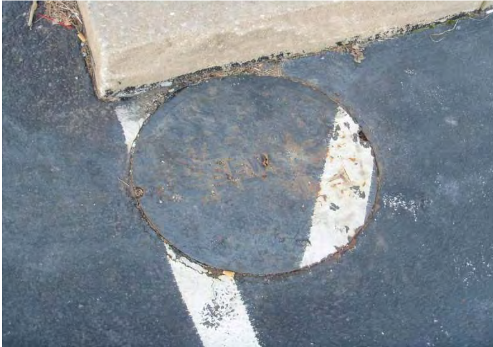
49. VIEW OF WASH WATER HOLDING TANK ACCESS POINT AT HANOVER NISSAN
