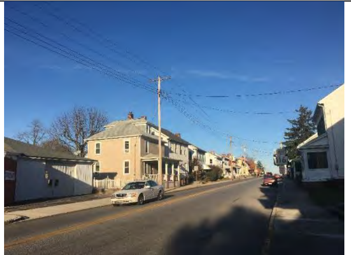
Looking northeast along Main Street from 2 nd Street.
