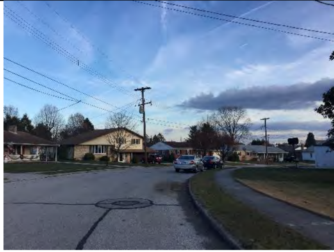
View looking southeast along Shafer drive, from east of the intersection with High Street.
