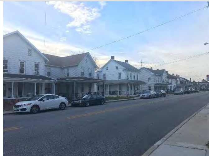
Key # 001966, looking northwest at the south side of 3 rd Street near the intersection at Washington Street.
