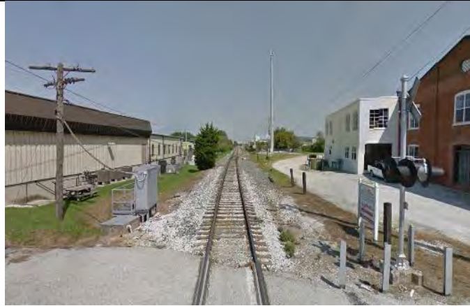
Looking north along the former Gettysburg Railroad, where it crosses Elm Avenue.
